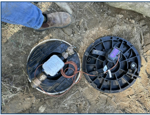
Finished installation of 3/4" meter in a meter pit.
