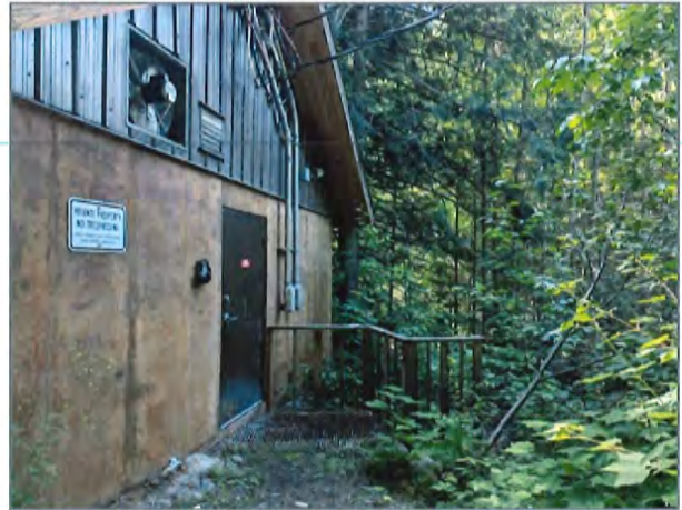
Photo 2. North side of powerhouse facing Dennis Creek (July 7, 2026).
