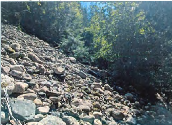
Photo 5. Penstock alignment within 30 m WDP area, section 2 (July 7, 2026).
