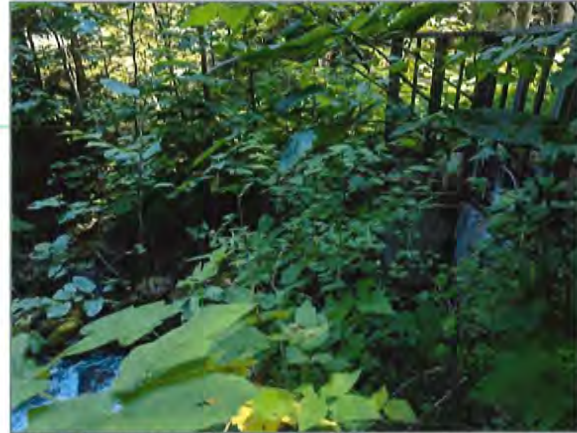
Photo 9. Outflow from powerhouse to Dennis Creek (July 7, 2026).
