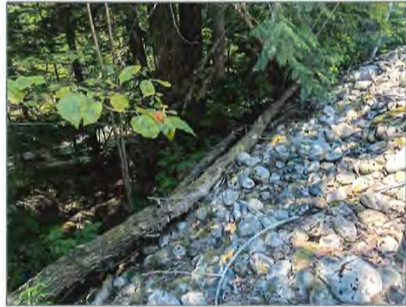
Photo 20. Toe edge of sloped section where additional logs will be placed (July 7, 2026).
