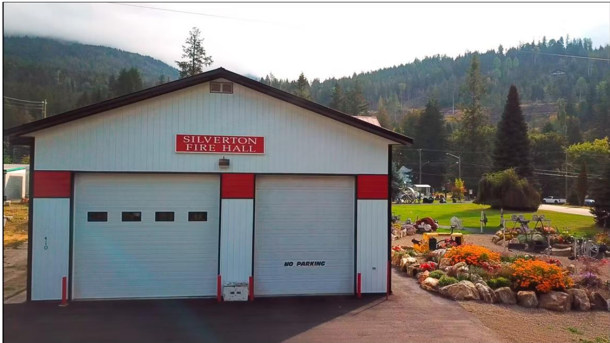
Figure 15. Silverton Fire Hall. Source: SIFCo website.
