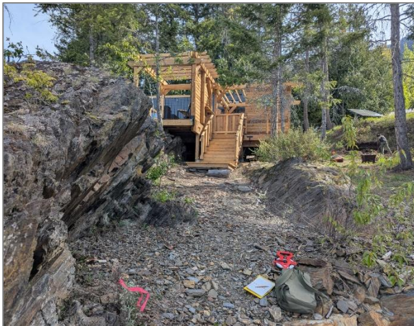
Photo 1. Deck structure within 15 m ESDP area (May 4, 2026).
