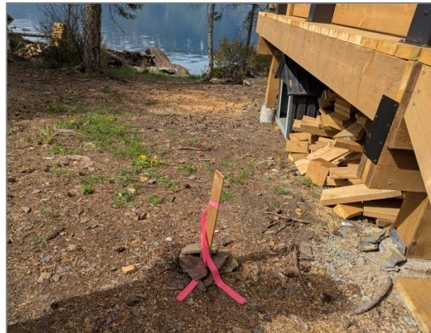
Photo 2. 15 m ESDP stake adjacent to deck structure (May 4, 2026).
