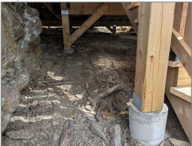
Photo 7. View under the deck where vegetation may have been removed (May 4, 2026).
