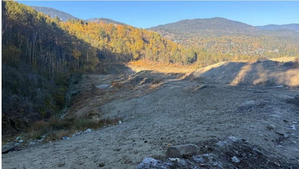
Figure 2: View of Slopes in Areas of High Methane Concentrations
