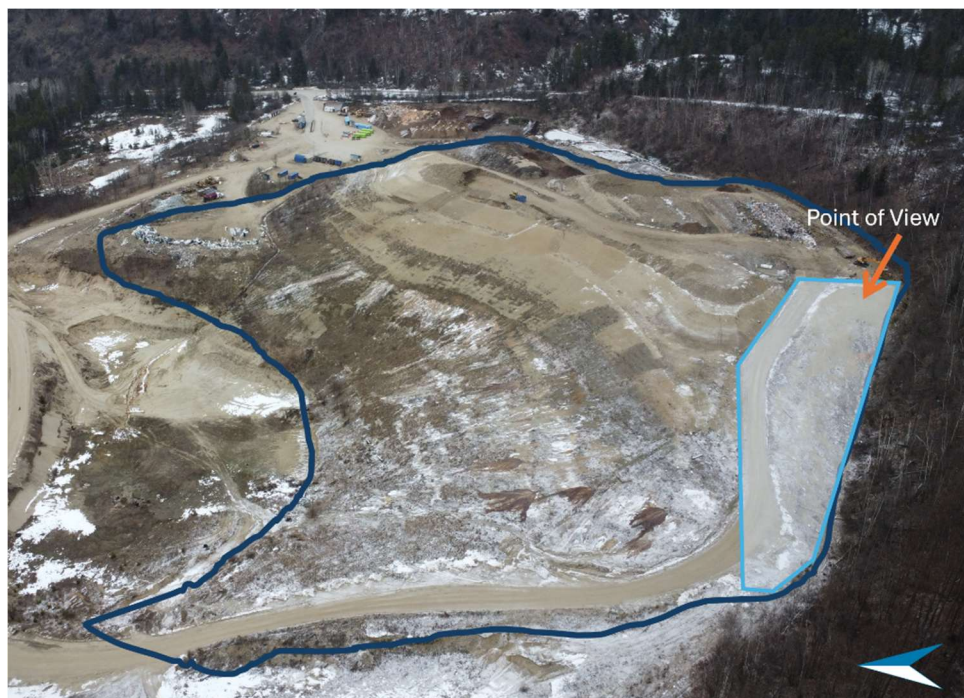
Figure 3: Area of High Surface Methane Concentrations at the Ootischenia Landfill
