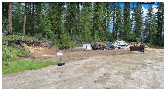
Site after cleanup
