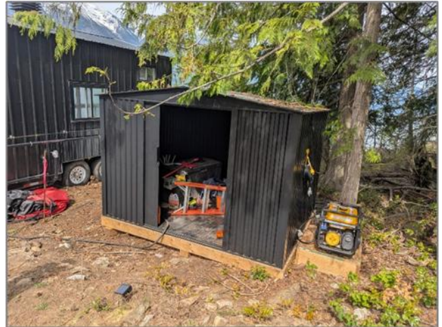
Photo 4. Shed partially within 15 m ESDP area (May 4, 2026).
