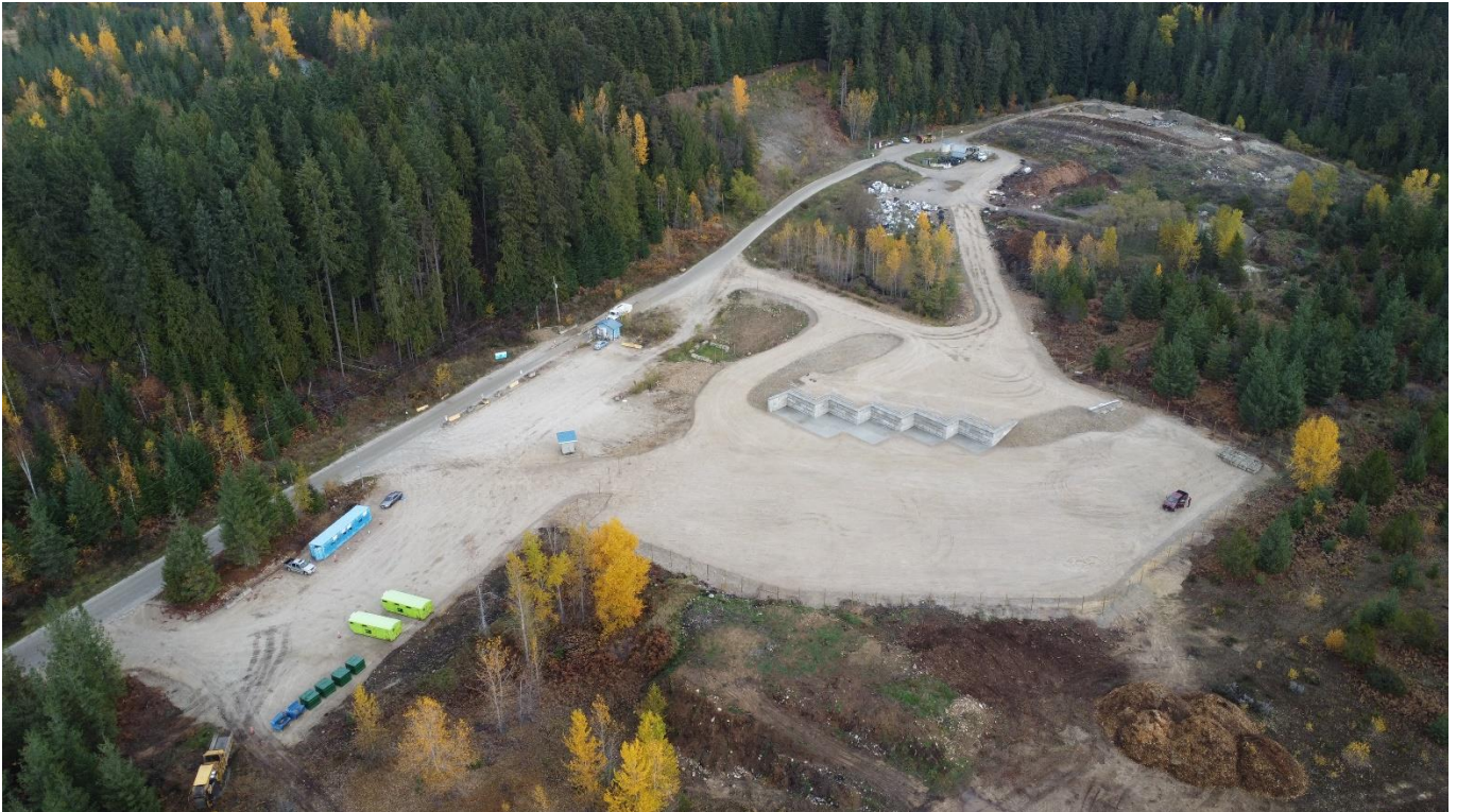
Photo 2-1: 2024 Nakusp Transfer Station Construction
