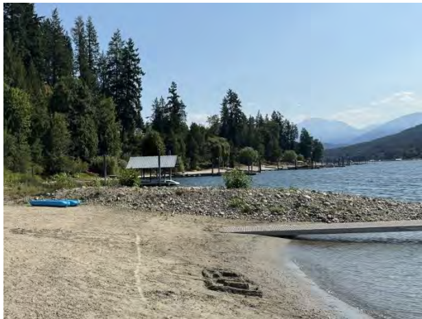
Photo 6. Existing groyne within Crown Land foreshore on the east side. Aug. 13, 2025.
