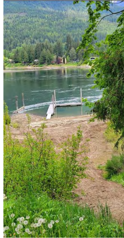
Photo 2. View of Site on Crown Land adjacent to Subject Property post unauthorized works. Photo provided by Alan Tite. May 2025.
