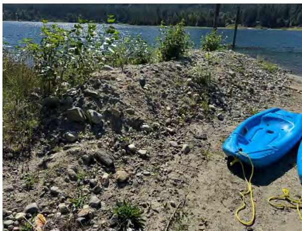
Photo 4. Mixture of cobbles, gravels and fines placed against existing east groyne. Aug. 13, 2025.
