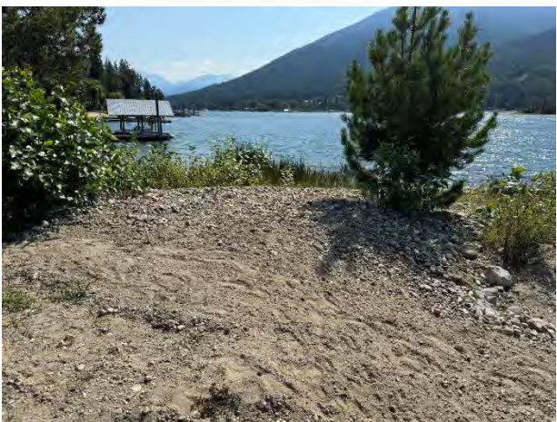
Photo 3. Mixture of cobbles and gravel placed at the upper end of existing east groyne. Aug. 13, 2025.
