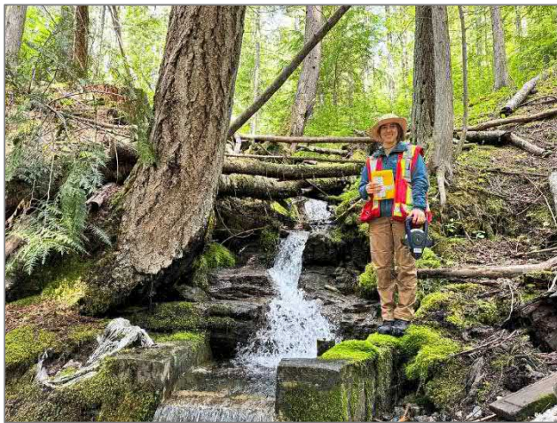
Photo 1. Water intake structure within 9201 Fisher Avenue on Ross Creek (June 2, 2026).
