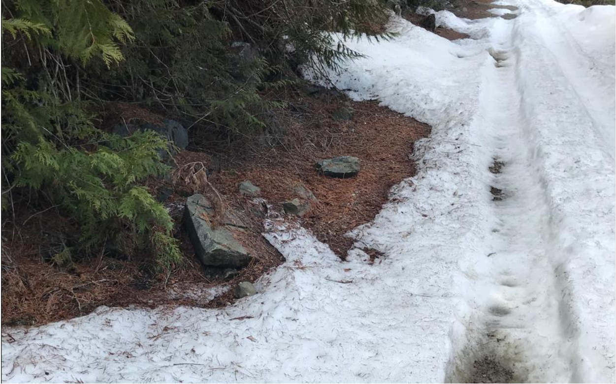
Figure 3. Photo taken April 4, 2026 showing a few rocks that would require moving.
