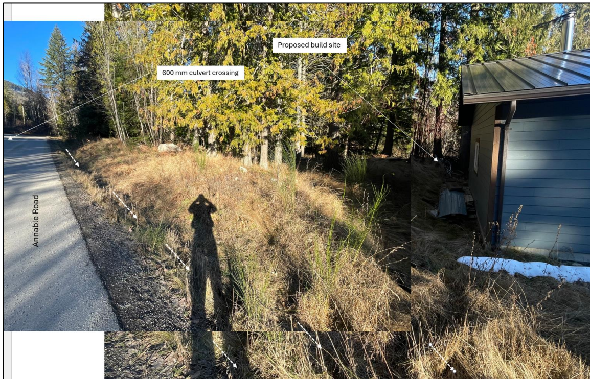
Photo 7: View looking at the Annable Road surface and ditch adjacent to the property. The white flow directional arrows indicate the path of overland flow from a blockage/ capacity exceedance at the 600 mm culvert crossing on Annable Road.
