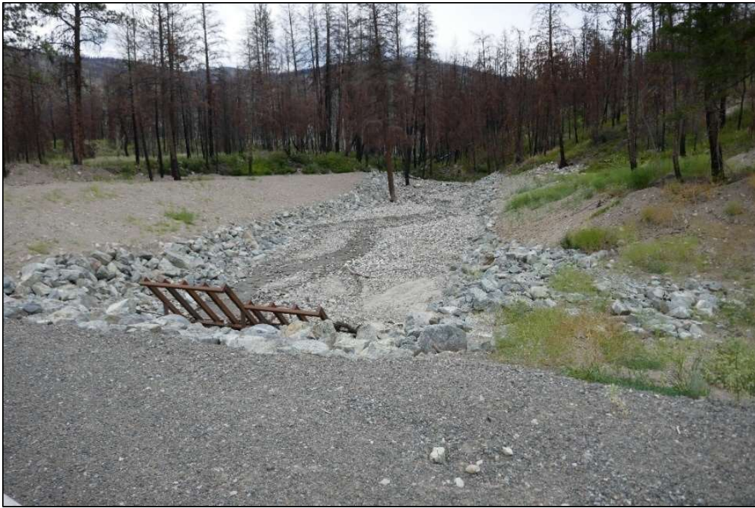
Photo 26: Construction of a wide channel through an armoured catch basin with a trash rack at the culvert inlet, such as shown in this image, may be a suitable solution at the highway crossing of Aylwin Creek.
