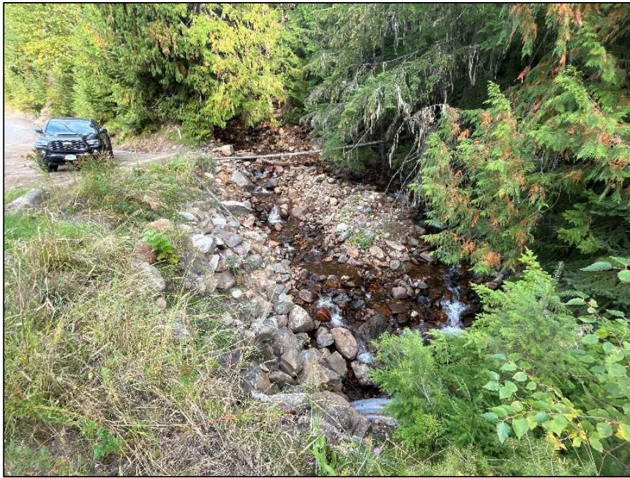
Photo 10: Looking upstream along Aylwin Creek from the Highway crossing (Field Observation Site K8). Note the low freeboard on the left side of the image where avulsion of the creek could easily occur and flow could be diverted onto the Highway.
