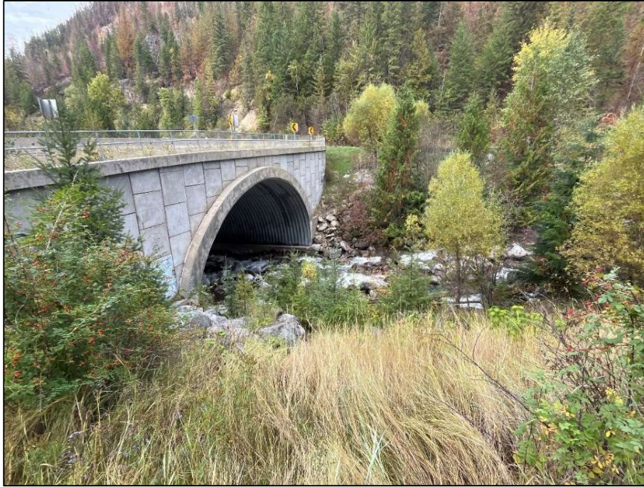
Photo 17: View of the inlet of the large arch culvert on Enterprise Creek at the Highway crossing (Field Observation Site K43).
