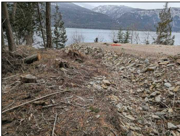
Photo 15. View of lower Bulmer Creek with armouring (Feb. 27, 2026).
