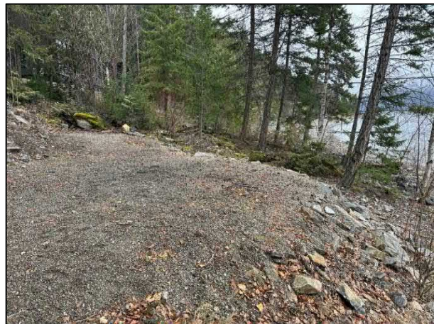
Photo 4. Bench south of access road within Lot 8 covenant (Feb. 27, 2026). Note large rocks used to armour bench.
