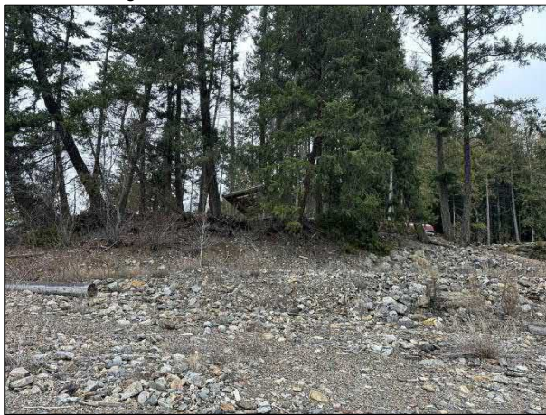
Photo 21. View of disturbed foreshore, access road and narrow strip of trees along bank (Feb. 27, 2026).
