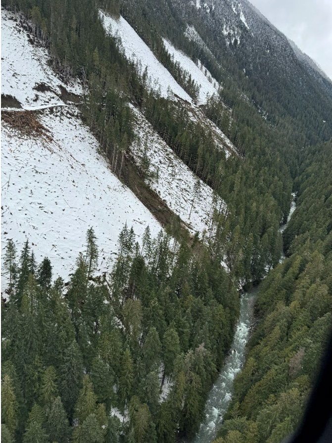
Photo 11. Landslides from forestry road.
