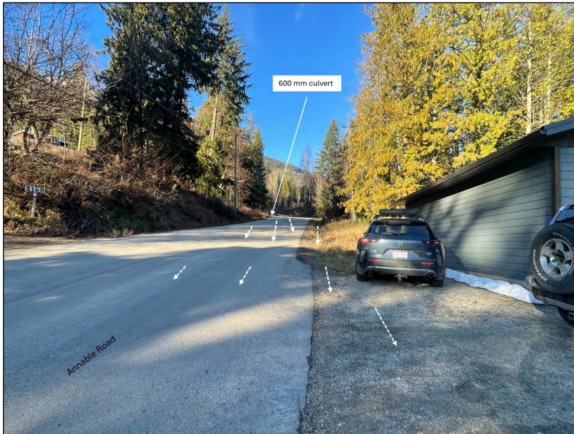
Photo 6: View of looking north along Annable Road at the location of the 600 mm culvert crossing from a vantage point on the west side of the property. The proposed build site is to the east or right side of the photograph on the east side of the garage. A culvert blockage or flow capacity exceedance during an extreme flood will result in water and debris flowing down the road (depicted by white flow directional arrows) bypassing the proposed build site on 2168 Annable Road. The road surface gradient is 10%.
