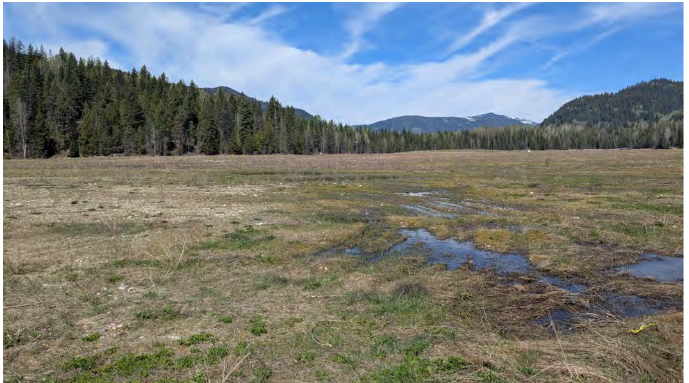
Photo 30: Area of ponding in the tailings pond backfill area. A review of the 2022 and 2025 cover surveys indicates no to minimal (i.e.. < 10 cm) differential settlement in the area.
