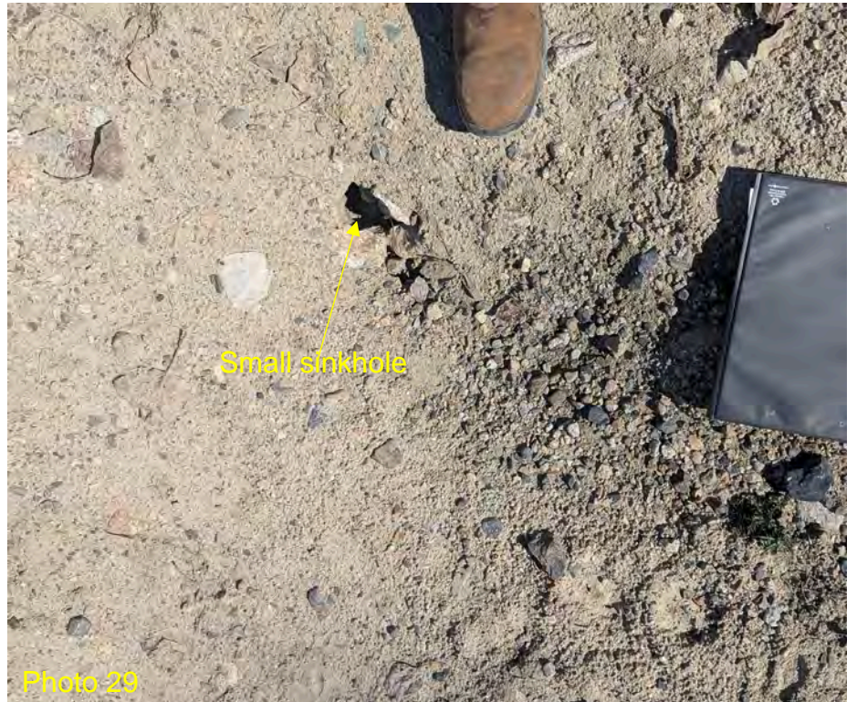
Photo 28 and 29: Small sinkhole on the toe berm crest near the east abutment caused by settlement of till into the underlying weighted filter. Approx 10 cm diameter; 15 cm deep.
