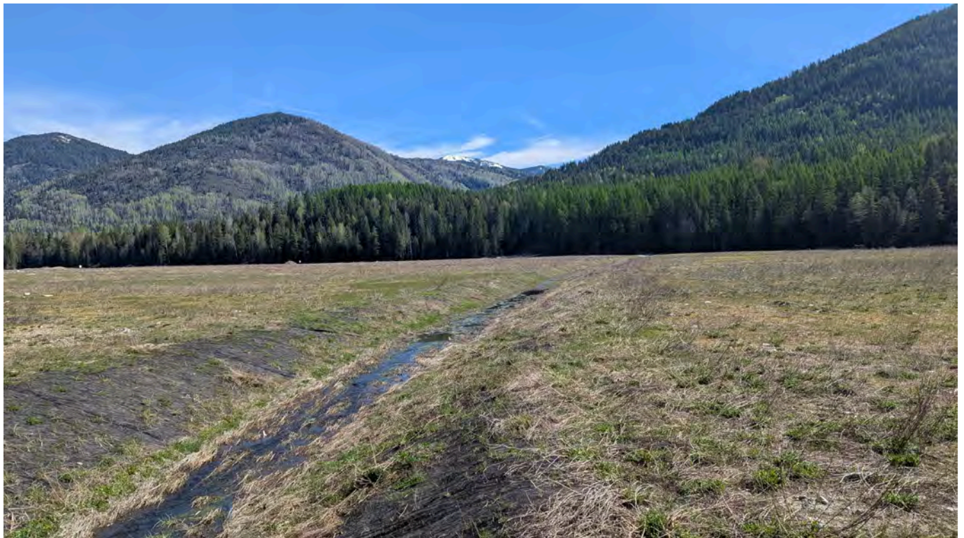
Photo 10: Main Tailings Surface Drainage Channel looking upstream from near the spillway inlet.
