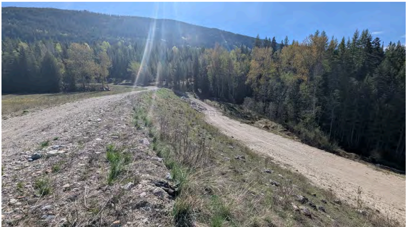
Photo 6: Dam crest and downstream slope looking east from near piezometers P1/P2.
