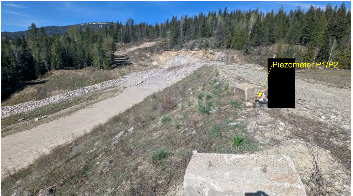
Photo 7: Dam crest and downstream slope looking west from near piezometers P1/P2.
