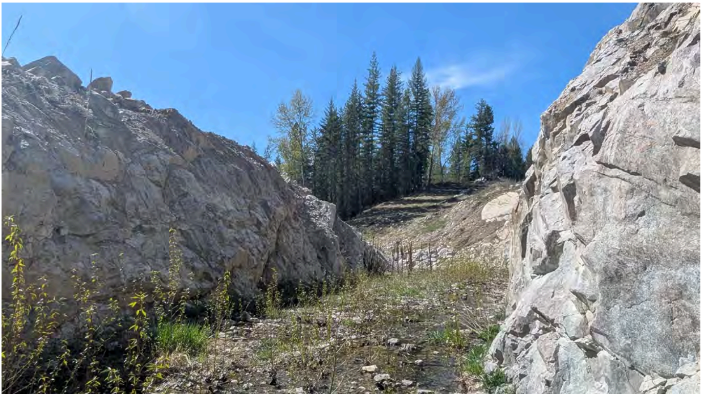
Photo 15: Bedrock spillway looking downstream.
