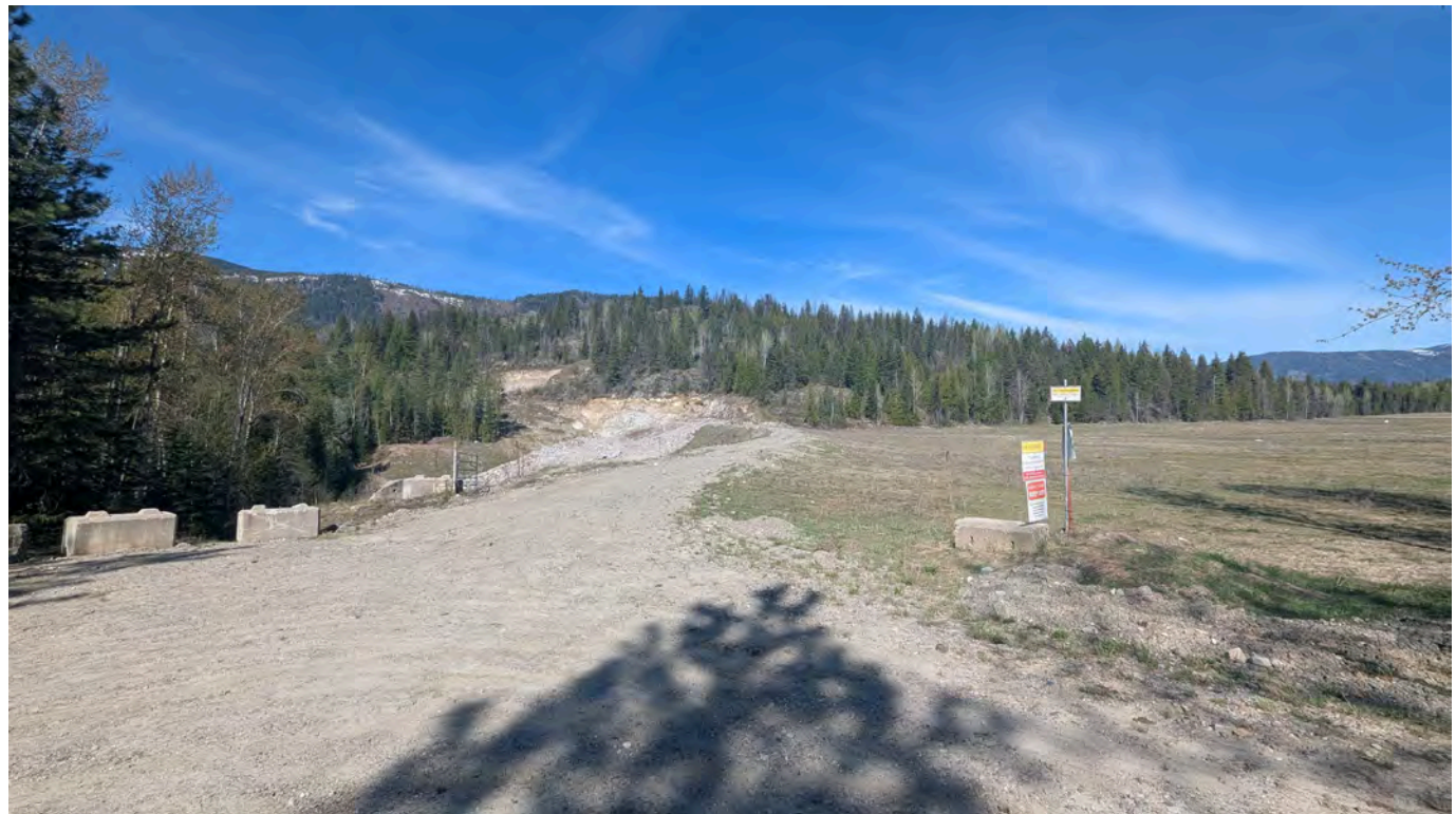
Photo 2: East abutment of the Dam crest looking west.
