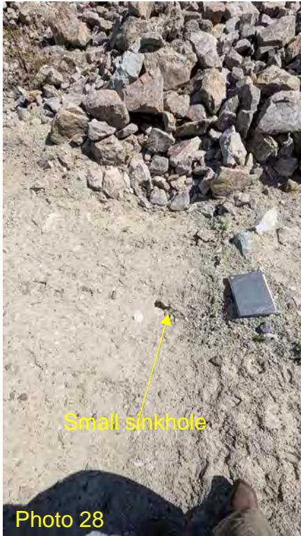
Photo 28 and 29: Small sinkhole on the toe berm crest near the east abutment caused by settlement of till into the underlying weighted filter. Approx 10 cm diameter; 15 cm deep.
