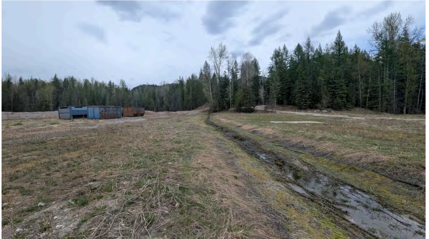
Photo 35: Main Tailings Surface Drainage Channel looking upstream.
