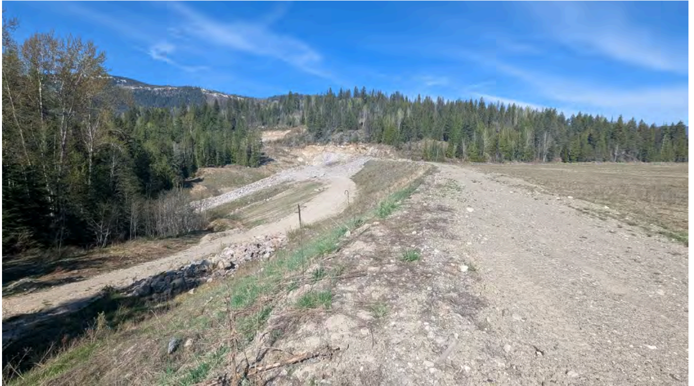
Photo 3: Dam crest and downstream slope looking west from the east abutment.
