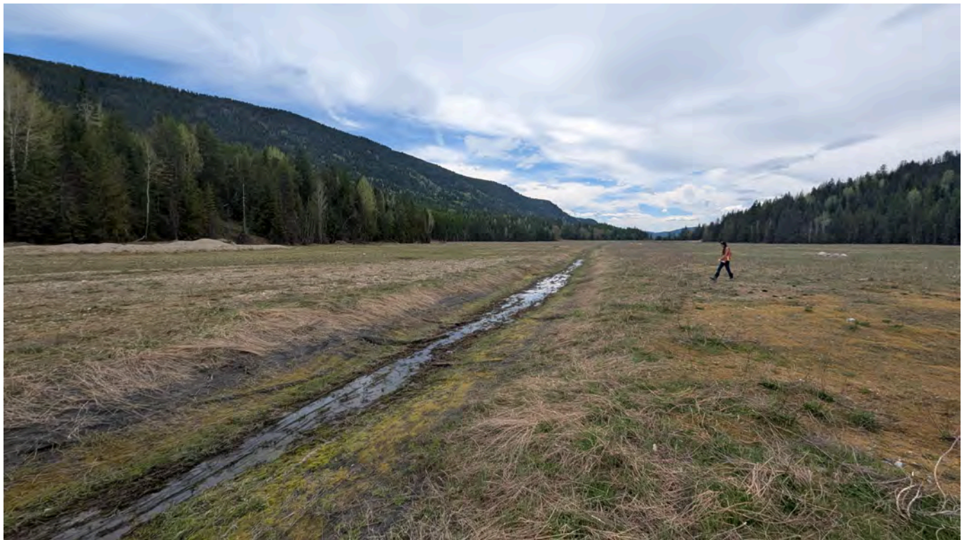
Photo 36: Main Tailings Surface Drainage Channel looking downstream.
