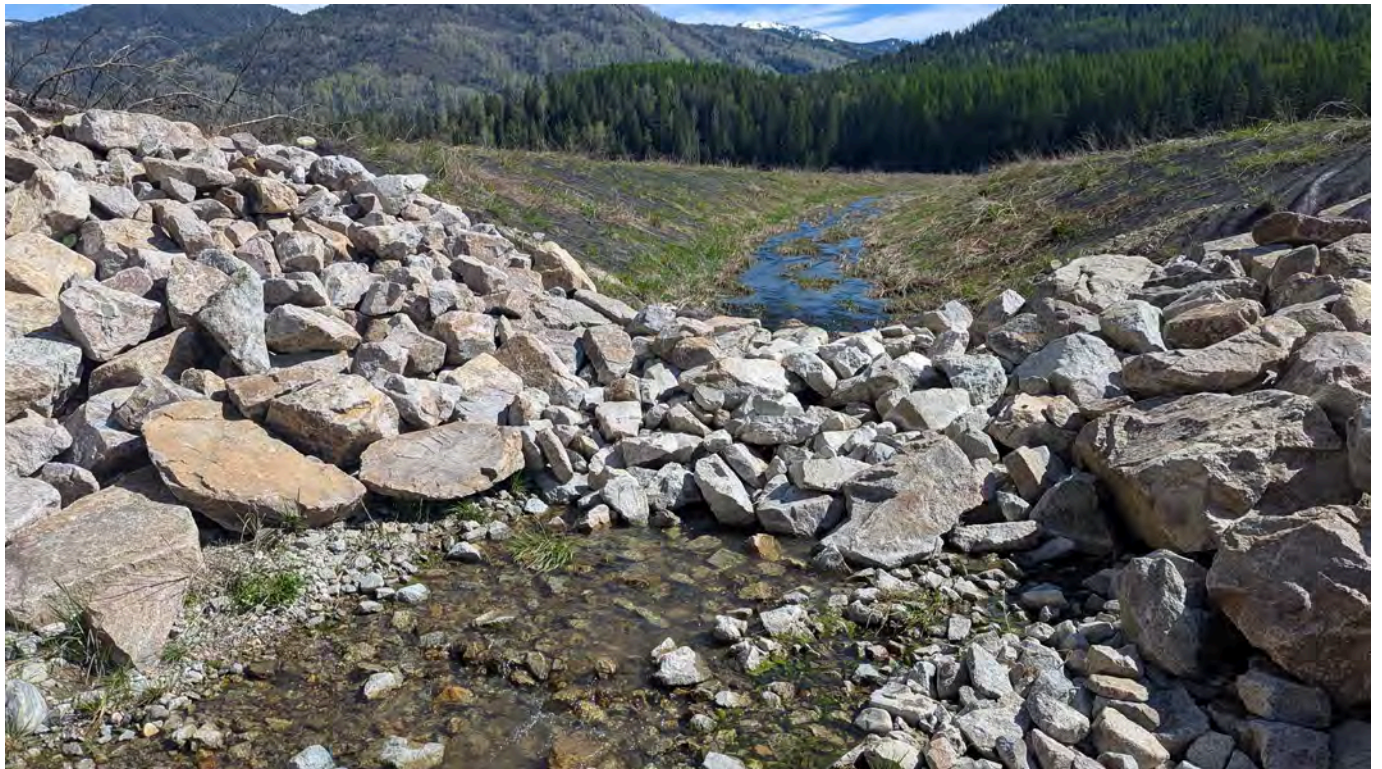
Photo 12: Riprap at the spillway inlet. No signs of riprap movement observed.
