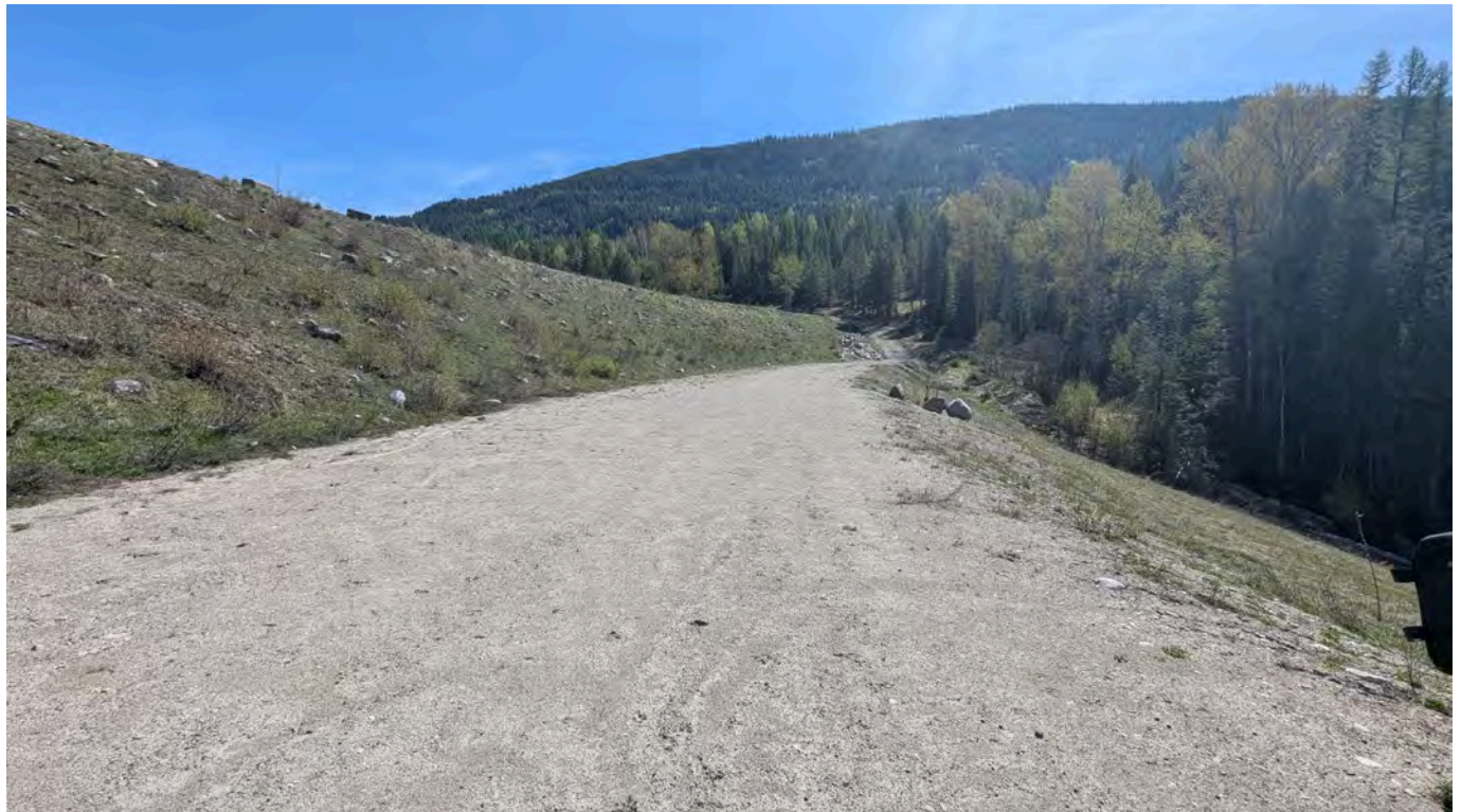
Photo 25: Crest of the toe berm looking east.
