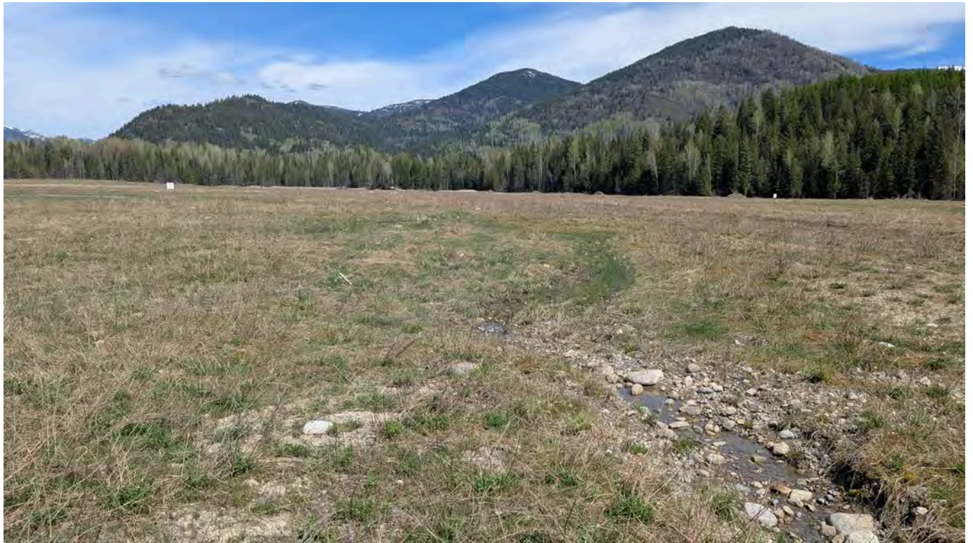
Photo 33: Small channel formed from runoff on the west side of the TSF looking north. Water flows parallel to the Main Channel and enters the Main channel near the spillway. No change compared to the 2024 inspection.
