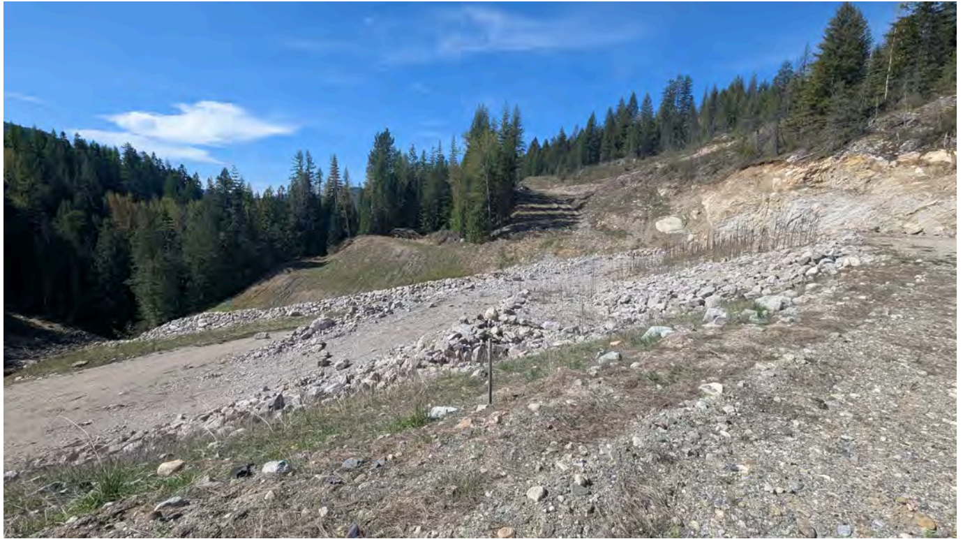
Photo 9: 2012 Blast Rock Repair area looking southwest.
