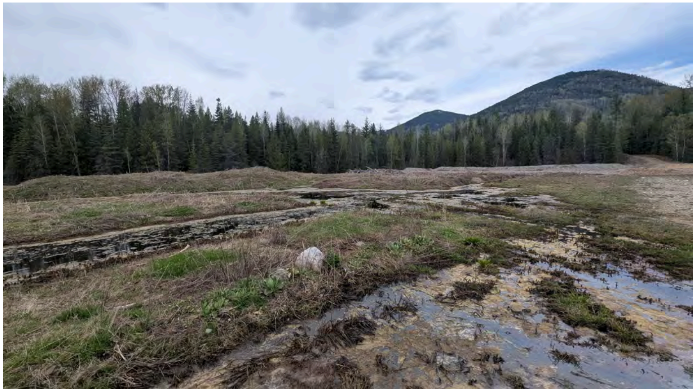
Photo 34: Small misc. stockpiles from the Central Landfill operations at the north end of the tailings impoundment. Several areas of ponded water are present with watering having a reddish colour.
