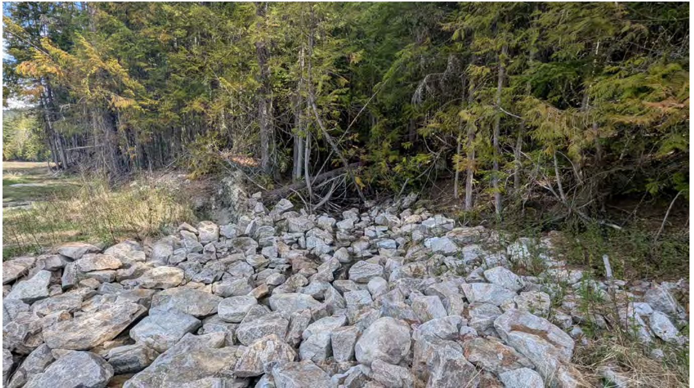
Photo 31: South Spur Channel Energy Dissipation Structure looking upstream.
