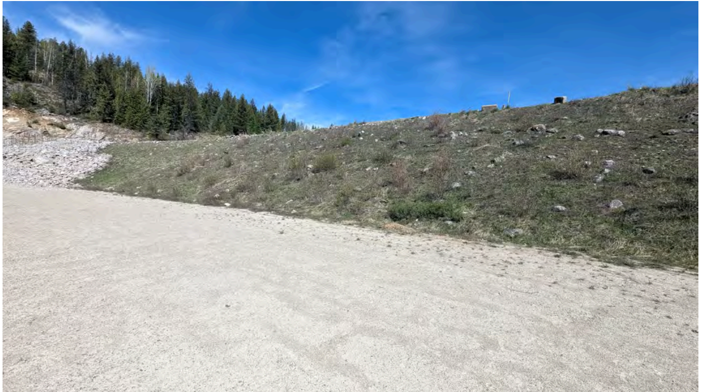
Photo 26: Downstream slope of the dam looking northeast from near piezometers P5/P6.
