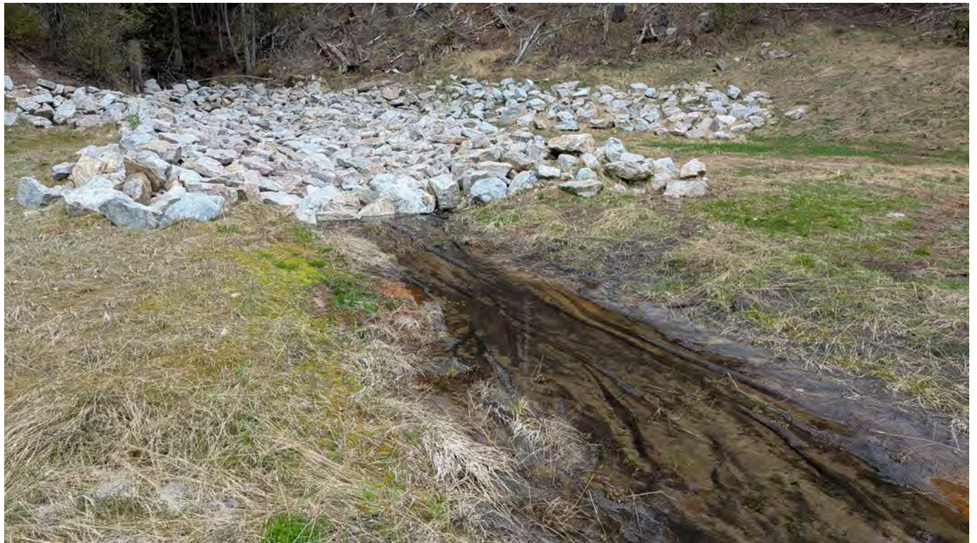
Photo 40: North Spur Energy Dissipation Structure looking upstream.
