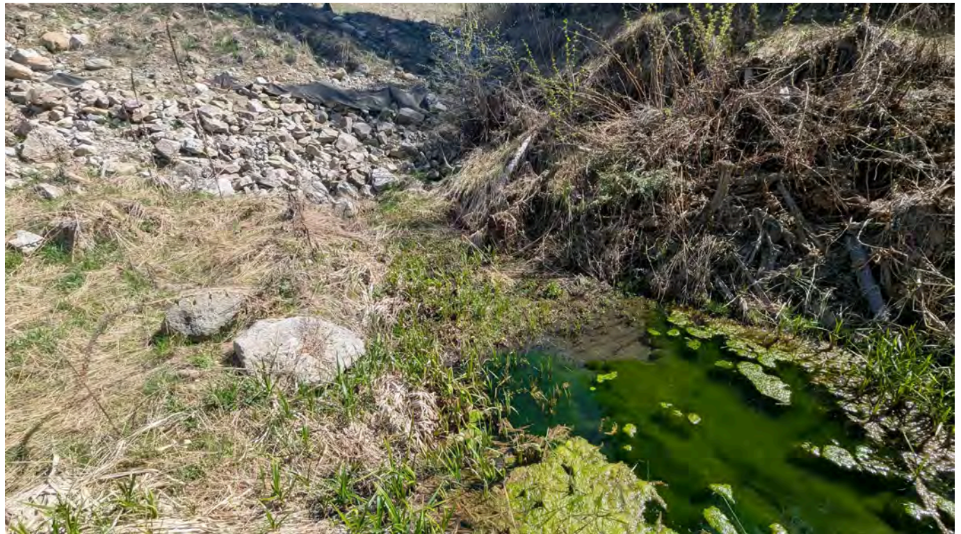
Photo 21: Area between the dam toe and seepage weir.
