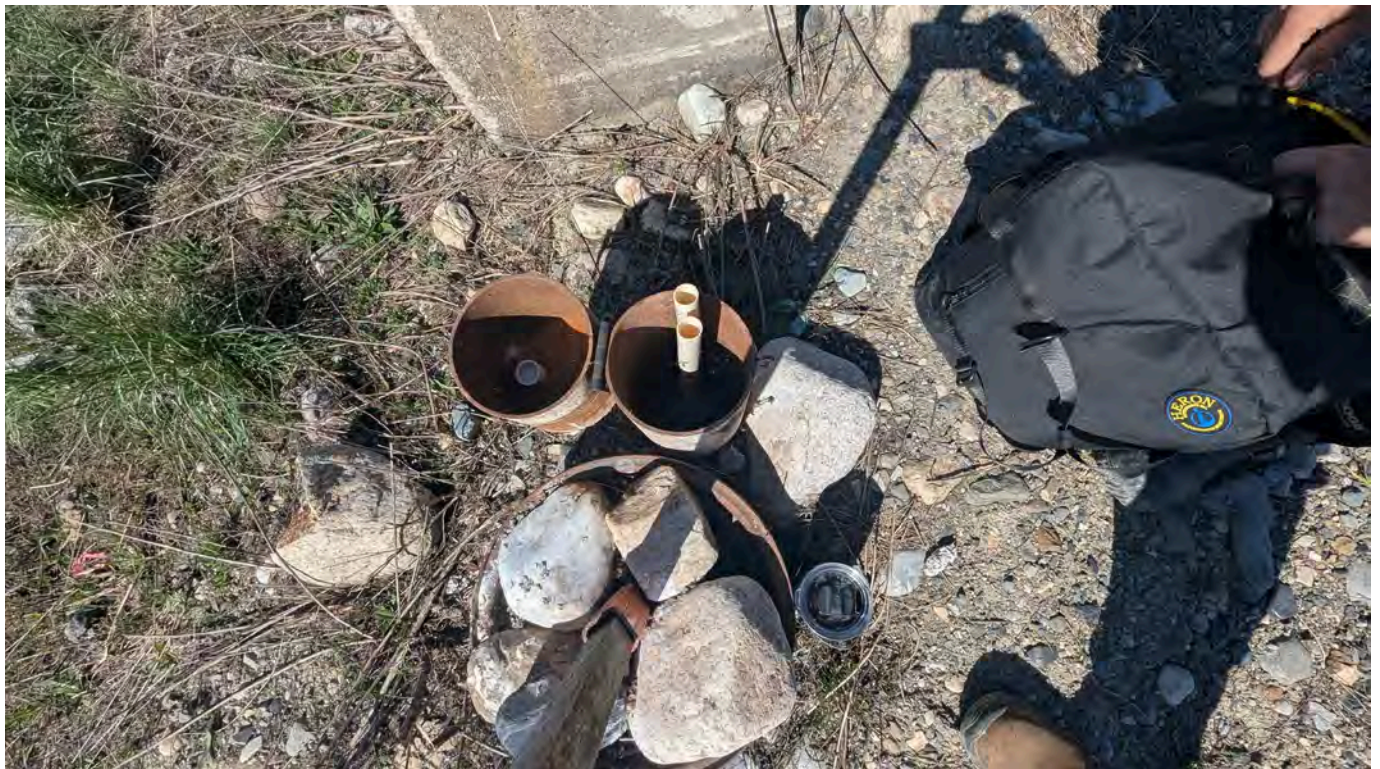
Photo 8: Piezometers P1/P2 at the dam crest.
