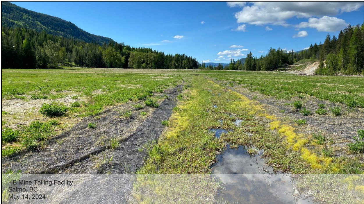
Photo D.33: General view of the upstream side of the dam, tailing impoundment area, and Tailings Surface Drainage Channel (Main Channel), looking south. Grassy vegetation is growing along most areas of the channels that needs to be monitored and removed.
