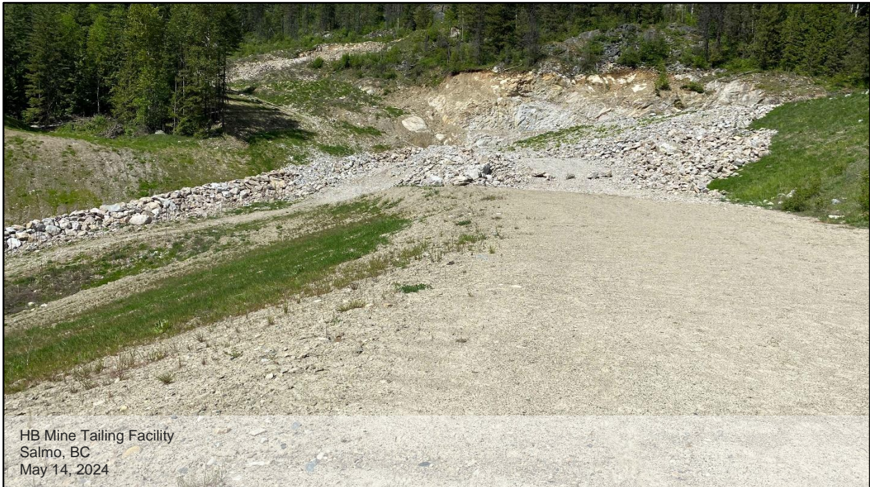
Photo D.21: General view of the crest and downstream slope (west side) of the expanded berm, looking west. The crest of the downstream toe berm was even and appears to be in general good condition.
