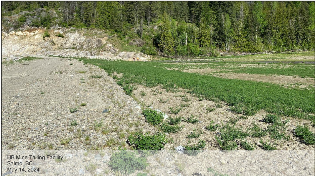
Photo D.7: General view of the tailing impoundment area, looking west. No sign/evidence of depression or sinkhole was noted along the interface with the tailing impoundment area.
