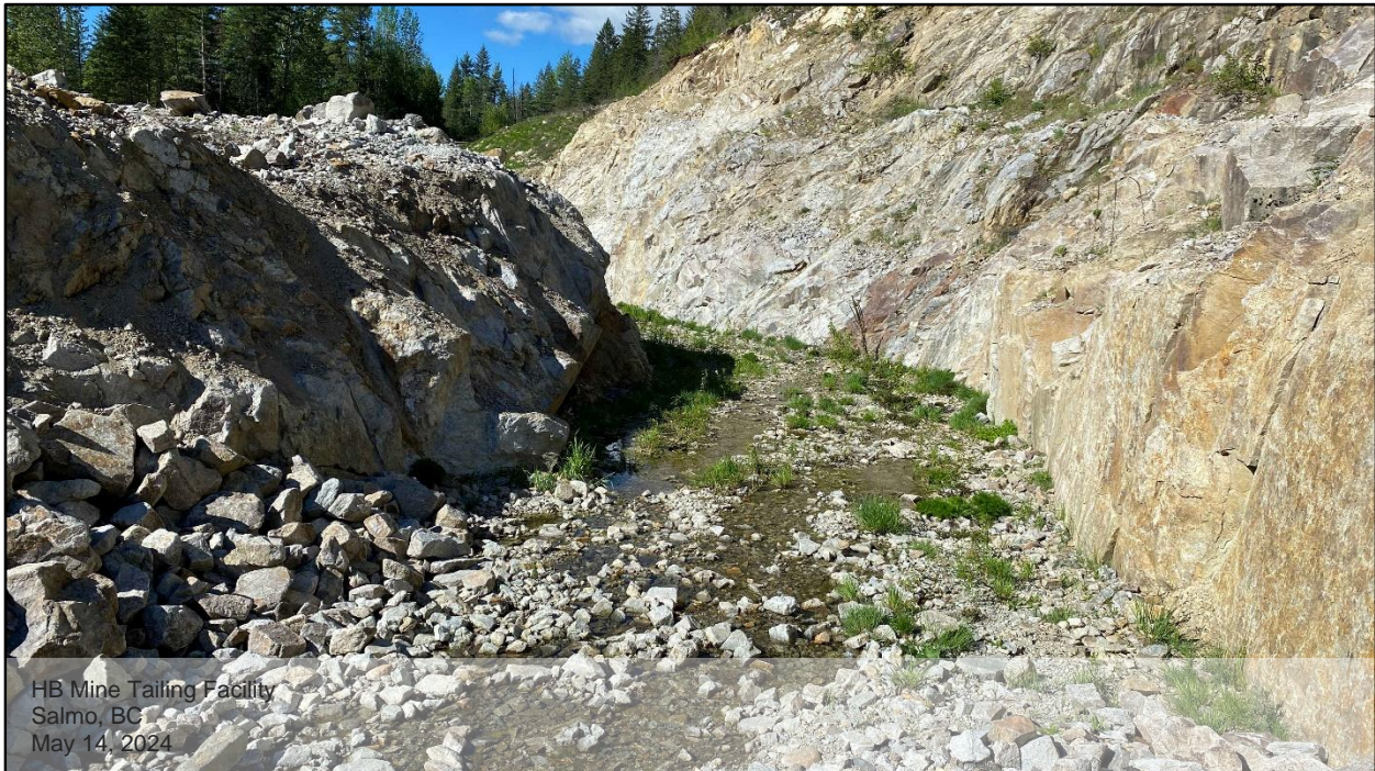
Photo D.11: View of the bedrock spillway inlet, looking south. Flow with a few centimeters' depth was observed over the bedrock spillway. Some vegetation is growing along the bedrock spillway.
