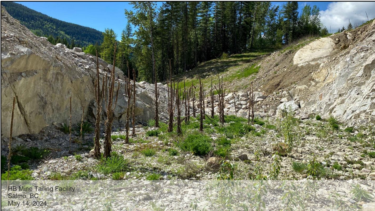
Photo D.13: View of the south end of bedrock spillway, looking south. Vegetation is growing along the bedrock spillway that needs to be removed.
