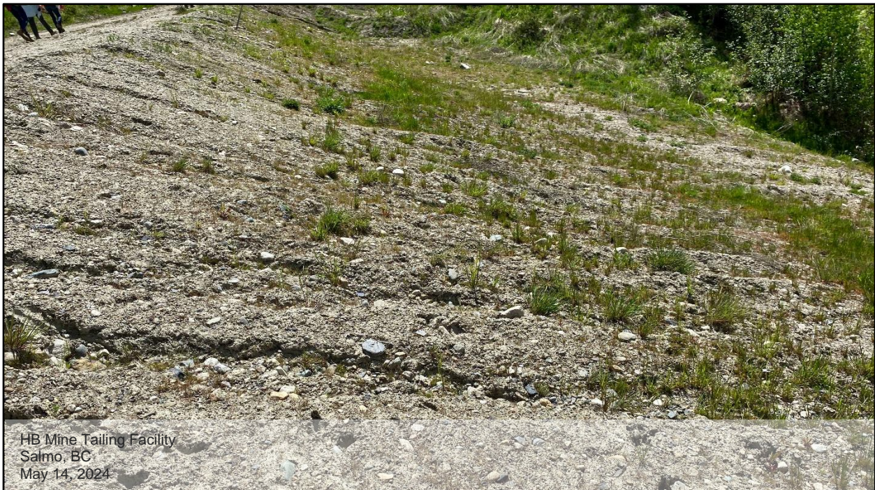
Photo D.22: View of the downstream slope (east side) of the expanded berm, looking east. Multiple surface erosion rills and gullies were identified along the eastern slope of the expanded berm.
