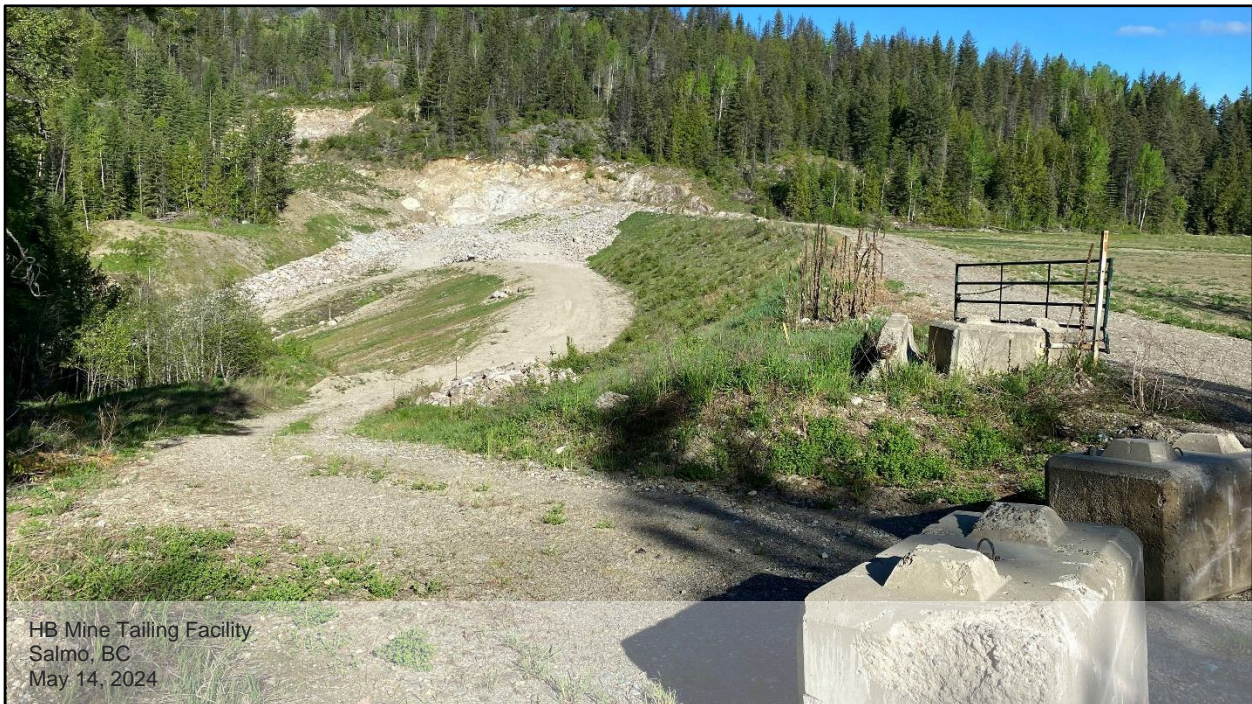
Photo D.2: General view of the downstream face of the dam and expanded berm from left (east) abutment, looking west. Access to the downstream berm from the left abutment was restricted by a couple of concrete blocks.
