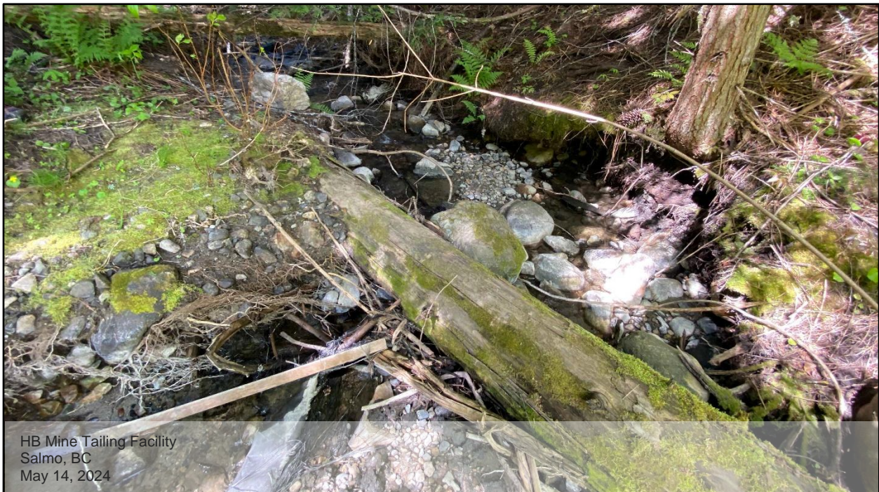
Photo D.18: View of the downstream creek, looking southwest. The seepage drains into the downstream creek (narrow valley). Logs and boulders were observed along the inlet of the downstream creek that need to be removed.
