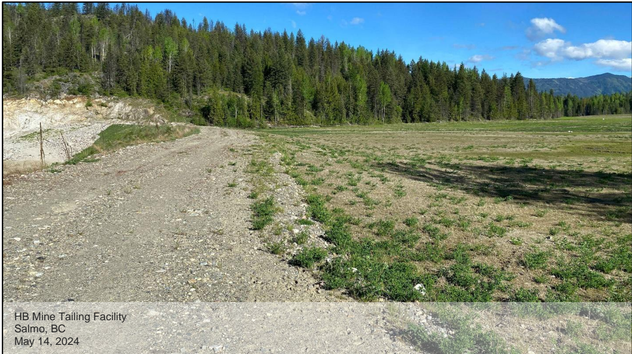
Photo D.3: View of the dam crest and tailings impoundment area, looking west. The dam crest was found to be mainly clean with no vegetation. The upstream slope of the dam has been covered by deposited tailing material, tailing cover, and vegetation growing over it.
