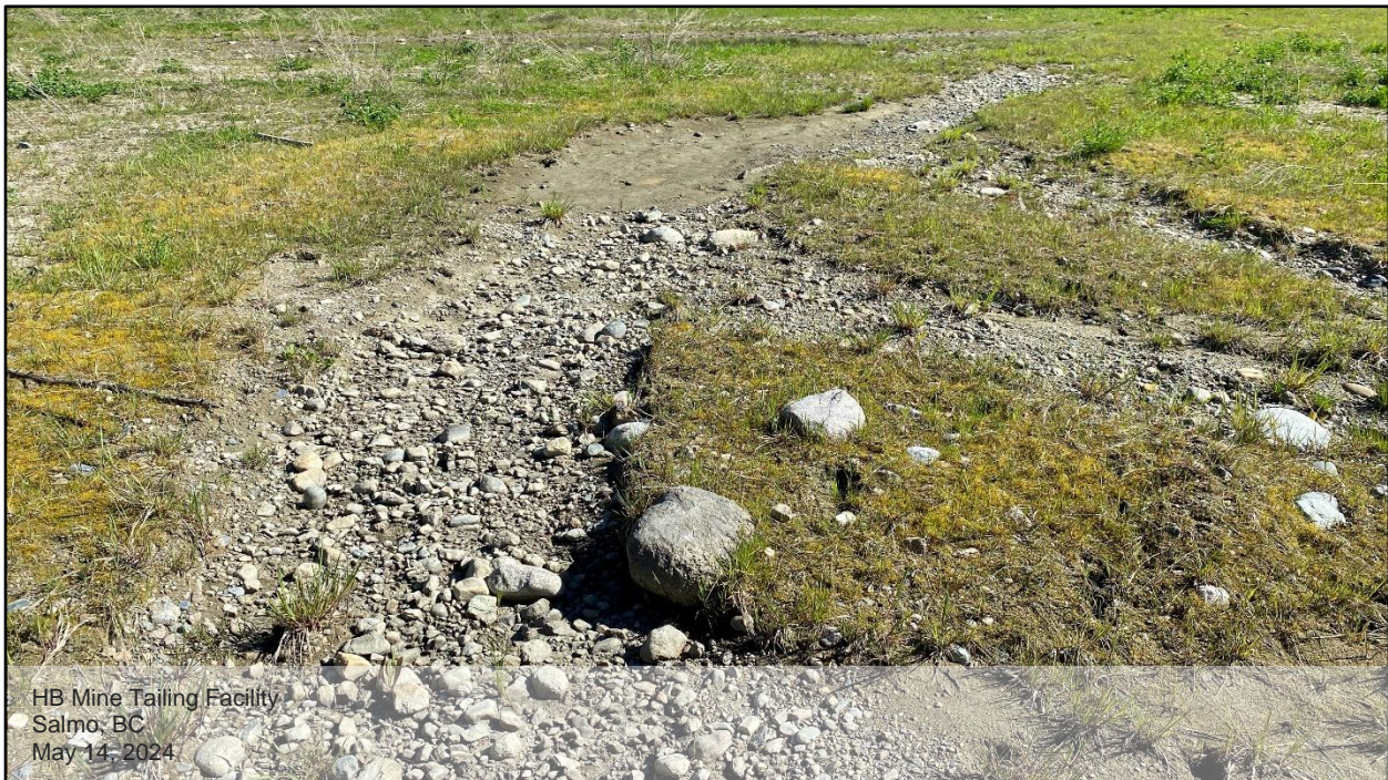
Photo D.26: Multiple surface eroded areas with several centimeters of depth were observed around the tailing cover perimeter.
