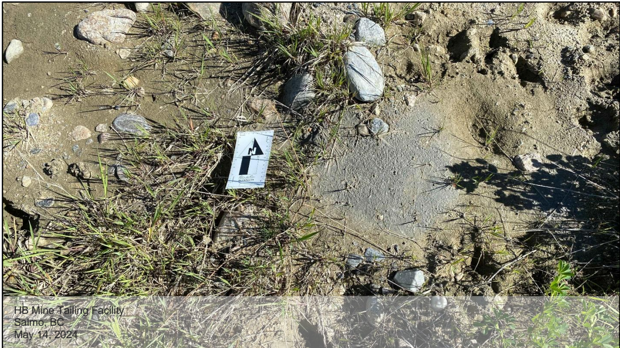
Photo D.27: A close view of the tailings exposure around the tailing cover perimeter.
