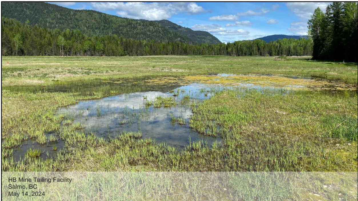
Photo D.28: General view of the tailing impoundment area, looking northwest. Water ponding and wetland areas were observed mainly along the east side of the tailing impoundment area.
