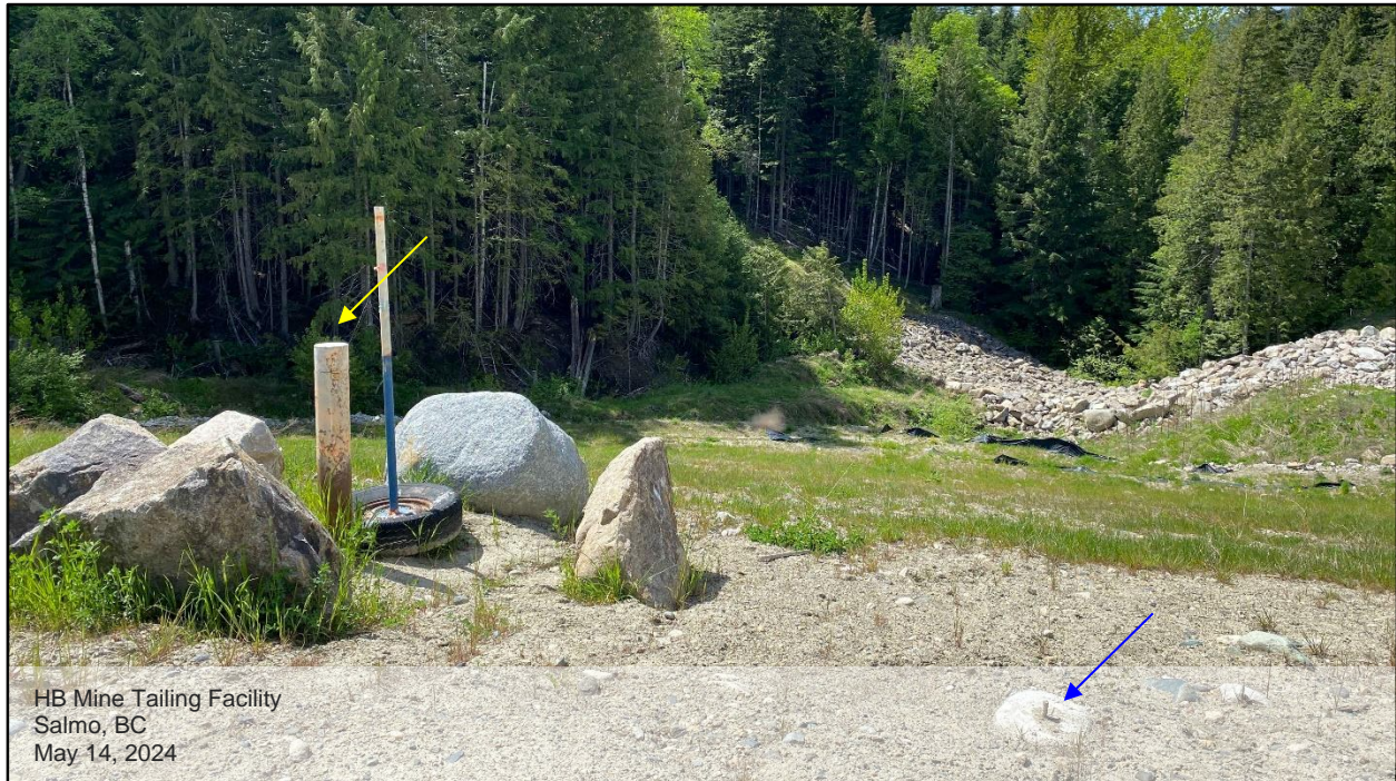
Photo D.19: View of the downstream slope of the expanded toe berm, looking south. Piezometers P5 and P6 (yellow arrow) and survey hub H11 (blue arrow) are located at the downstream slope of the expanded berm.
