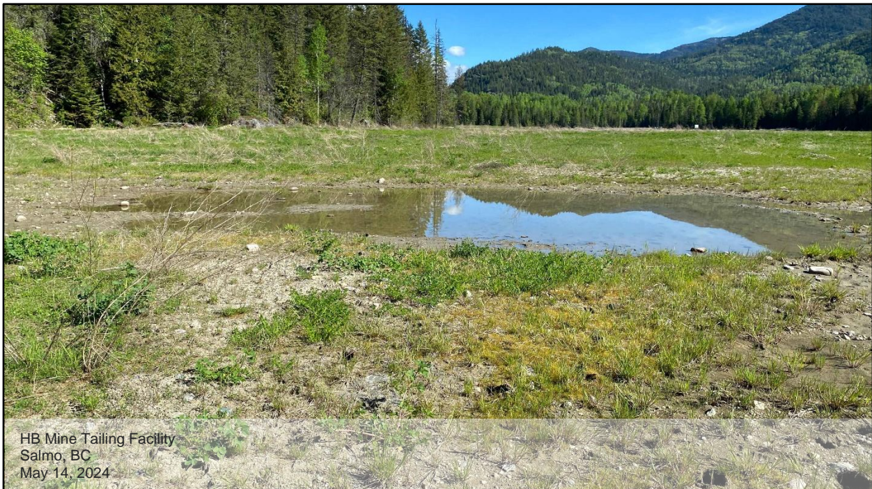
Photo D.34: Water ponding within the west side of the tailing impoundment area, looking north.
