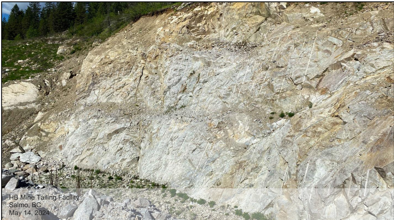
Photo D.12: View of the western slope of bedrock spillway. This area is visually inspected during the routine site inspections for any potential instability.
