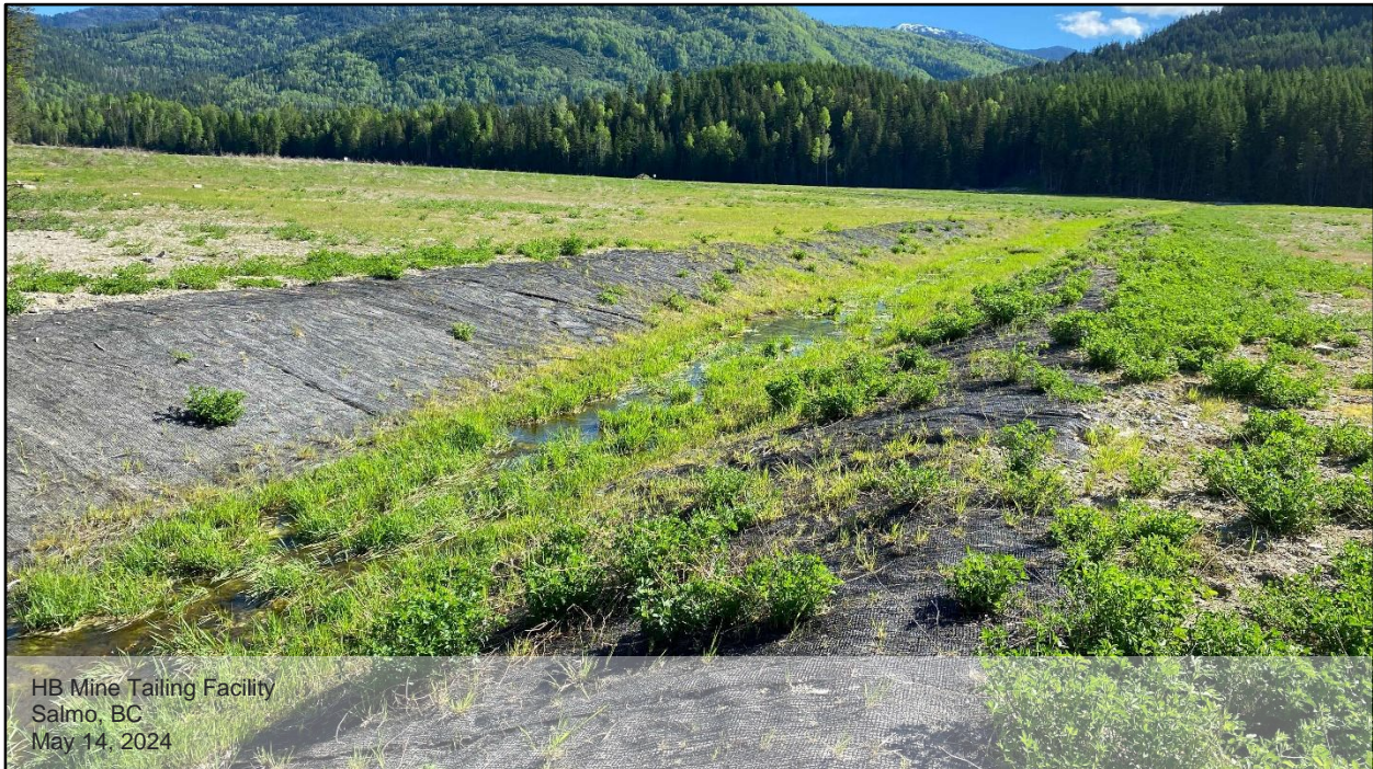
Photo D.25: General view of the tailing impoundment area and Main Channel, looking northeast. An erosion control blanket has been placed throughout the bottom and slope of the channels.
