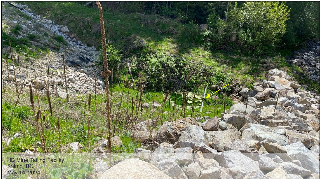
Photo D.17: View of the downstream toe, looking east. A seepage V-notch weir (yellow arrow) situated at the downstream toe of the expended berm measures the dam seepage flow rate manually. The seepage water at the downstream toe was clear with no turbidity.
