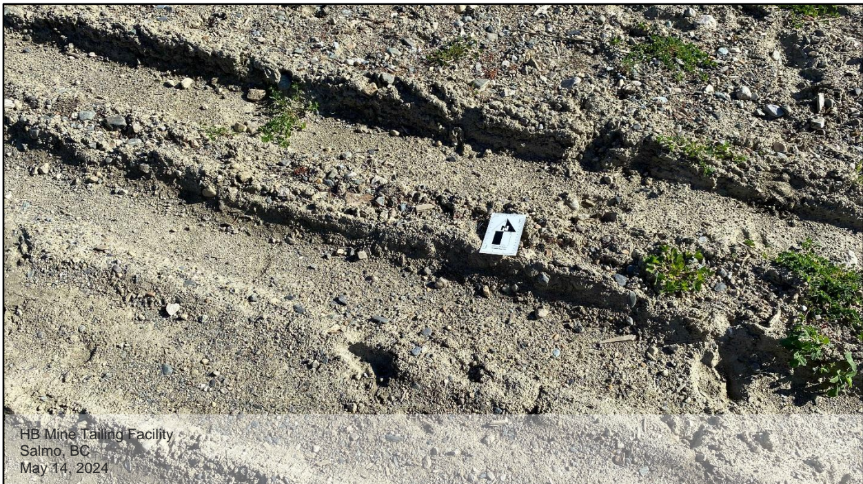
Photo D.4: A close view of the dam crest. Some rutting from vehicle traffic was observed along the dam crest. The dam crest is in general good condition.
