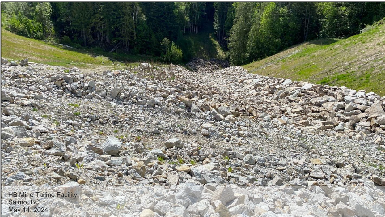
Photo D.14: View of the spillway outlet channel, looking south. The spillway channel appears to be in general good condition.
