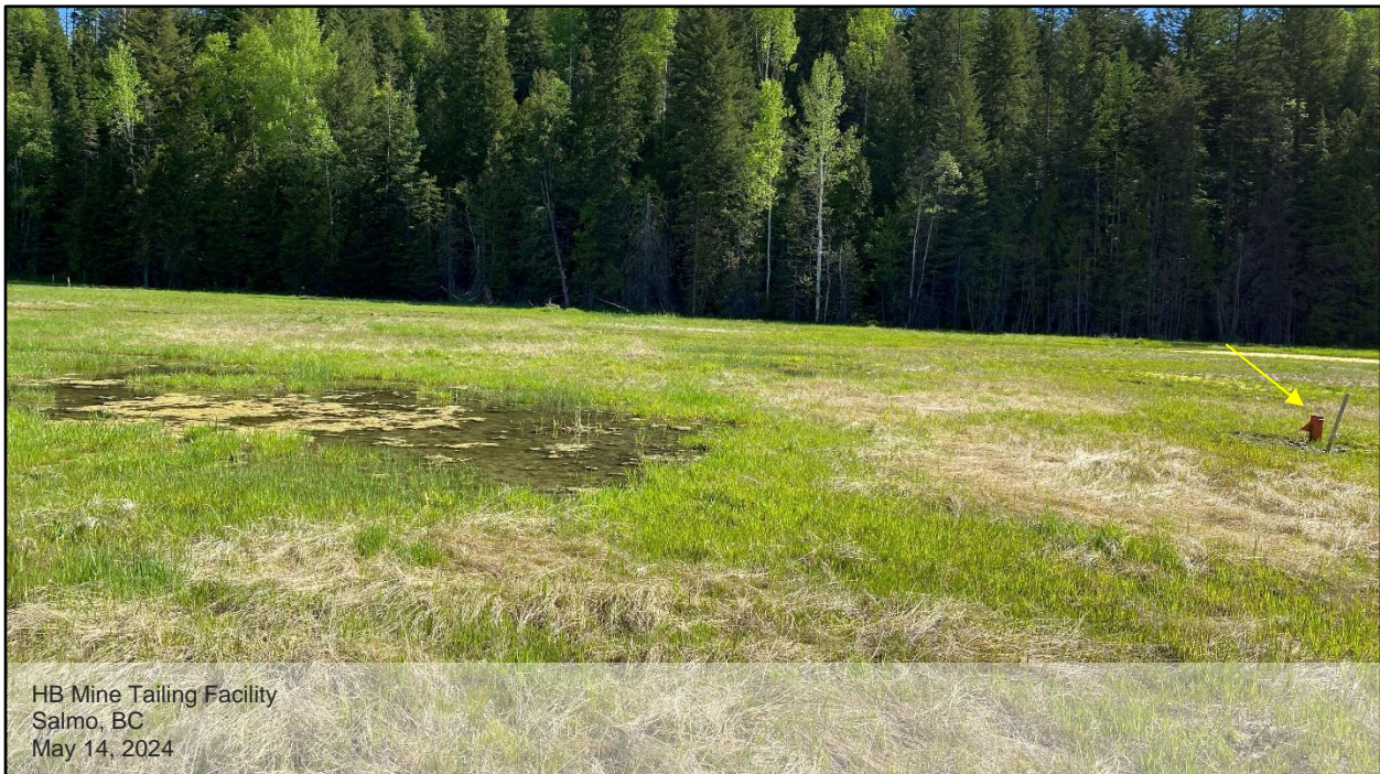
Photo D.32: View of the tailing impoundment area, looking east. A water ponding area was found near the monitoring well MW-04-S-05 (yellow arrow).
