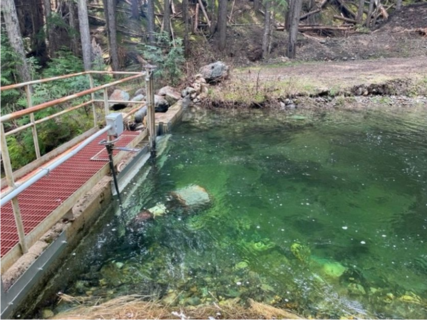
Figure 3-14 Quartz Creek Intake in Ymir
