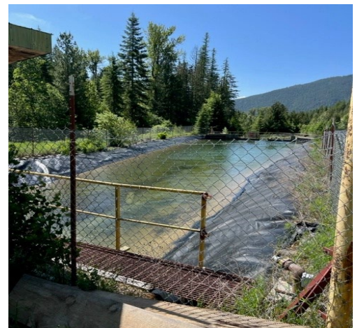
Figure 3-5 Settling Pond Arrow Water Treatment Plant
