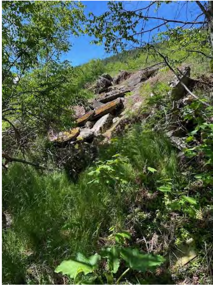
Photo 17: Debris visible on East edge of site, within steep slopes.
