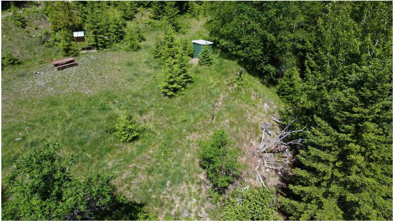
Photo 9: Pit Toilet with exposed waste and steep slopes noted at bottom right of photo.
