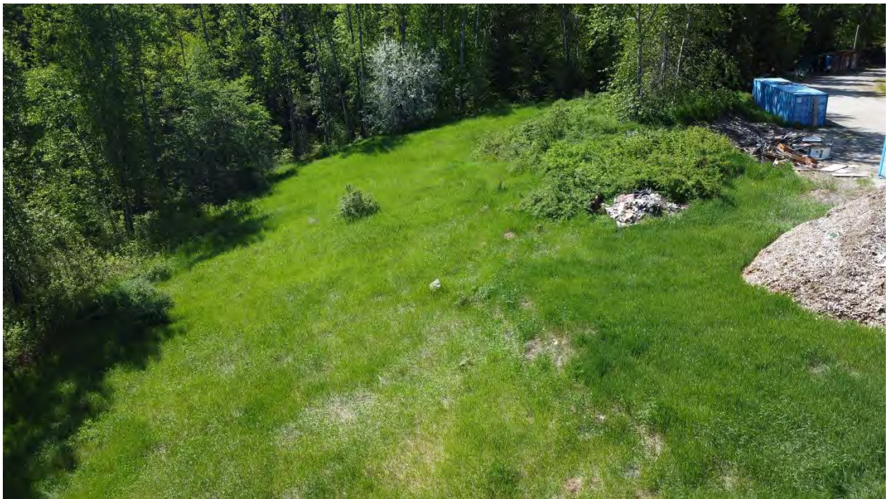
Photo 6: Taken from North side of landfill slope area, looking South.
