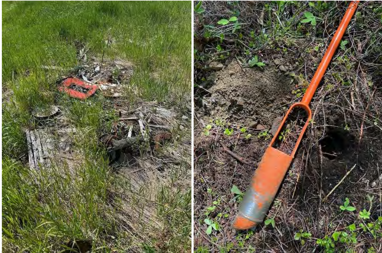
Photos 1 and 2: Exposed Waste on Landfill Area and Typical Cover Soil Found on Site
