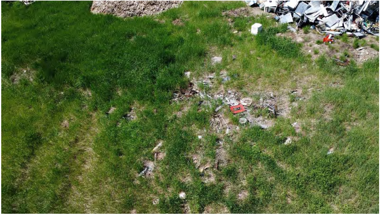
Photo 7: Exposed waste on landfill slope area.
