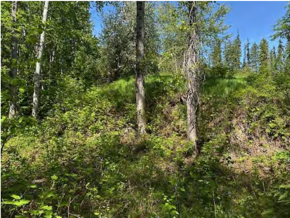
Photo 23: Bottom toe of landfill slope, viewed from historical perimeter road.
