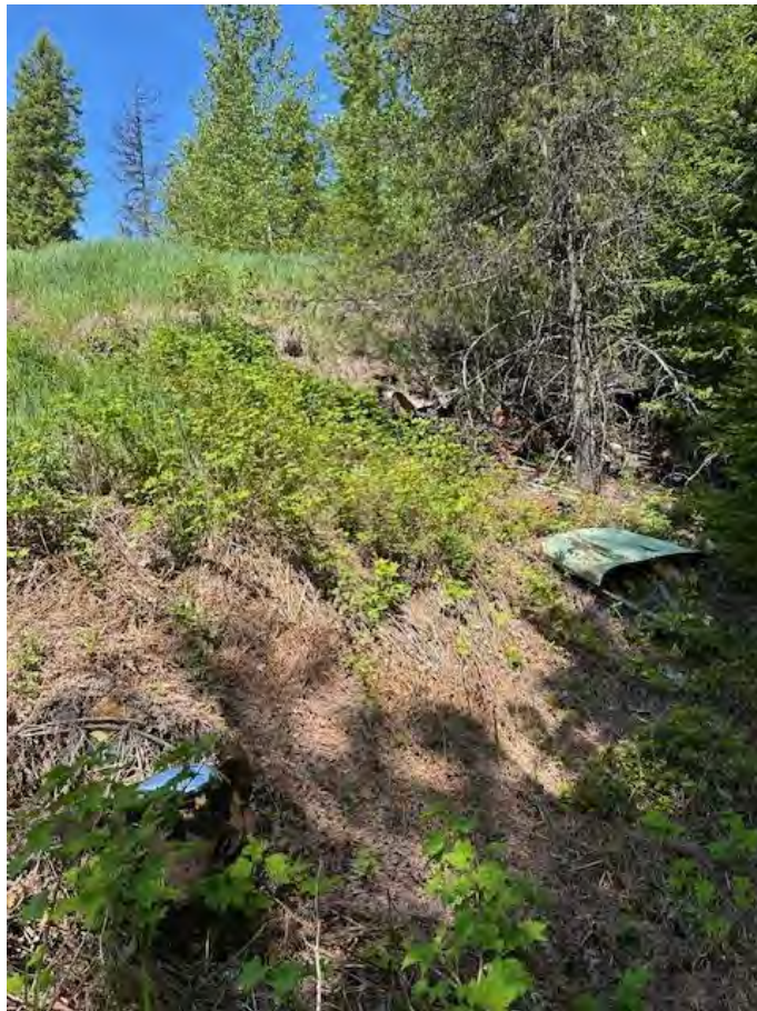
Photo 22: Steep slopes and exposed waste on North side of site, viewed from below.
