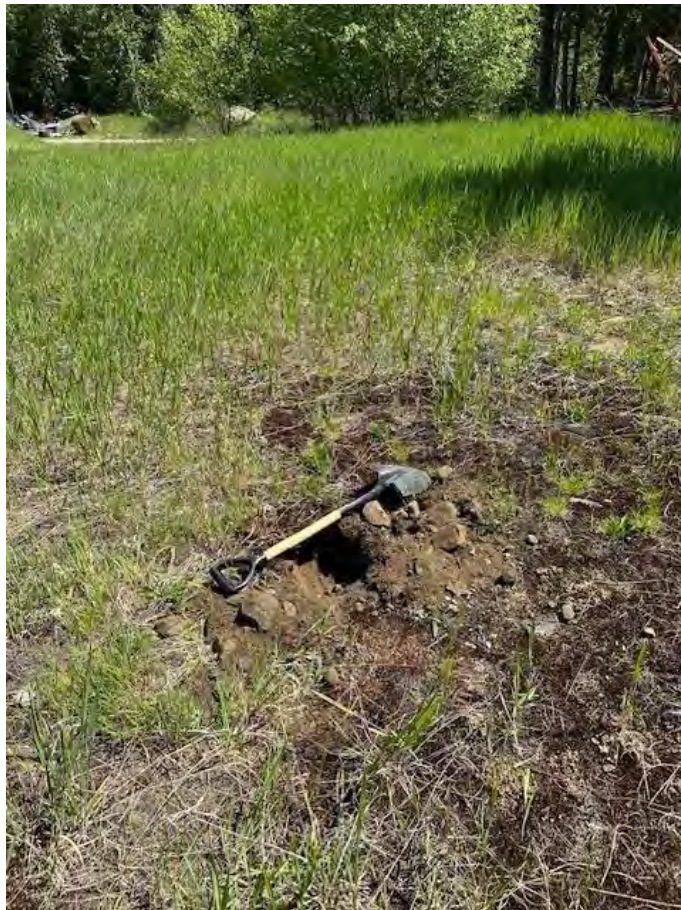
Photo 8: Cover investigation location 1 in Southern portion of site.
