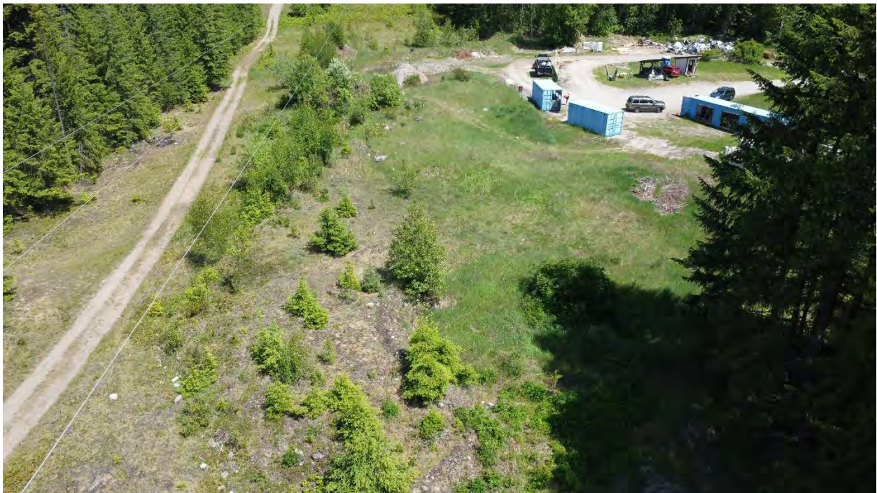
Photo 4: Landfill area with signs of settlement noted while on site.
