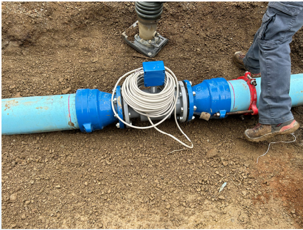
2024 District outflow meter installation
