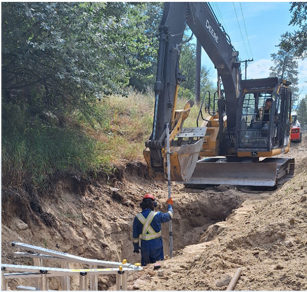
Phase 1 of the PN02 mainline replacement in 2025
