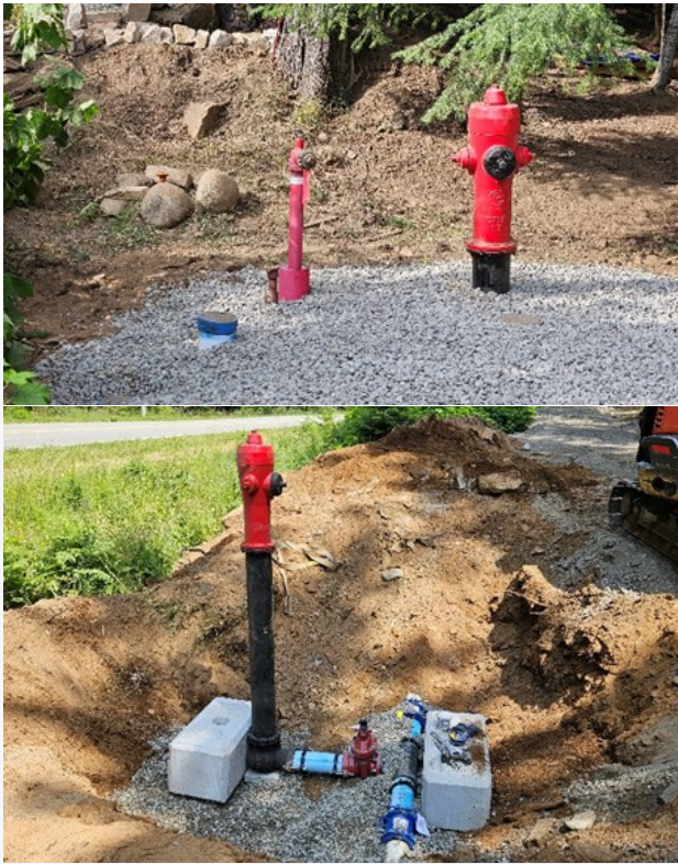
Fire hydrant installation 2025
