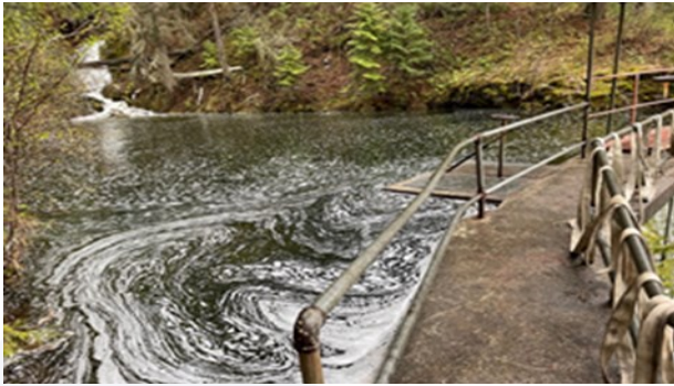
Smokey Creek Dam
