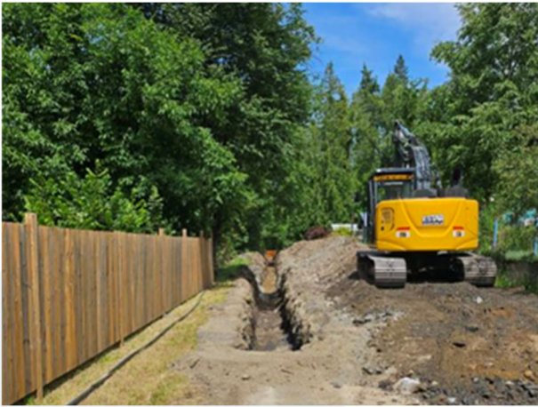
Ainsworth Ave mainline installation 2025
