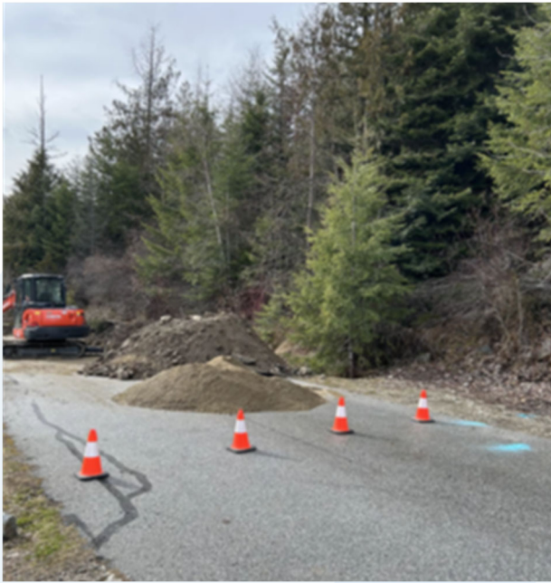
Mainline leak repair 2025
