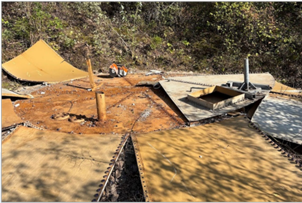
Old reservoir demolition 2025
