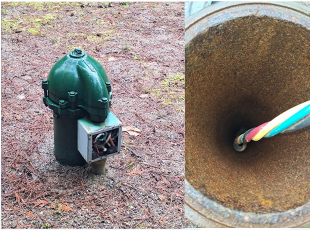
Well pump replacement 2025
