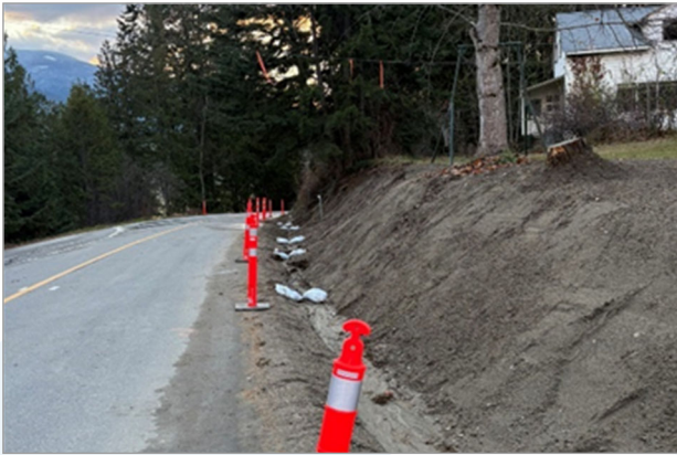
Upper Balfour Rd mainline replacement project 2025
