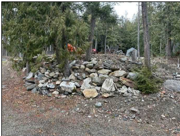
Photo 3. Erosion protection south of access road (Feb. 27, 2026).
