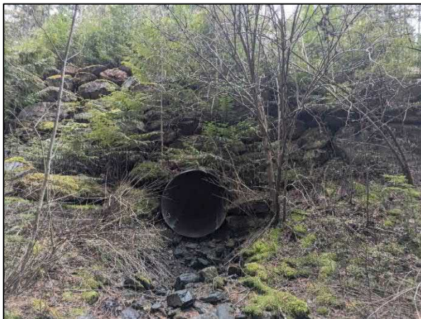
Photo 13. Culvert (1400 mm) under Bulmer Drive (Feb. 27, 2026).
