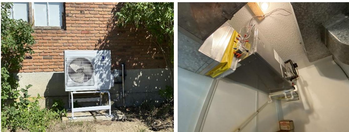
Figure 7: Air Source Heat Pump Outdoor and Indoor Units
