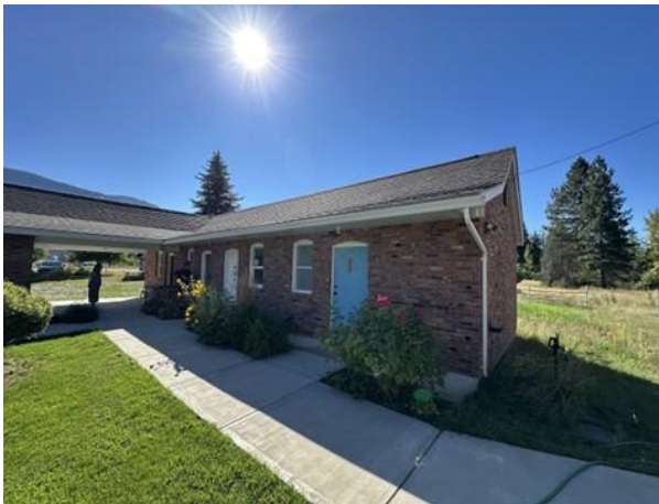
Figure 2: Exterior Photo of the South Annex Building
