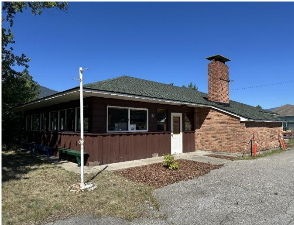
Figure 10: Exterior Photo of the Bistro Building
