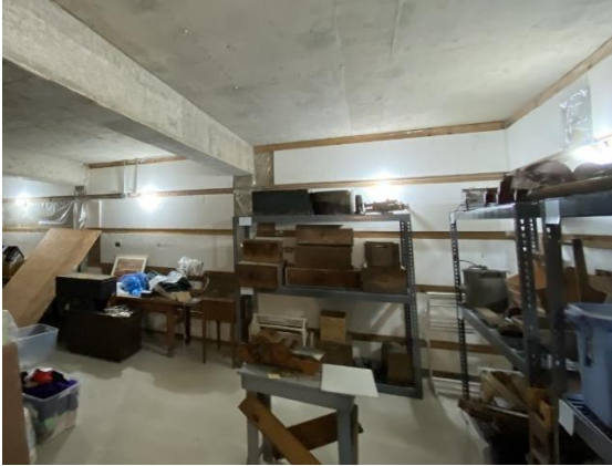
Figure 9: Interior Photo of the Basement Showing Partially Insulated Walls
