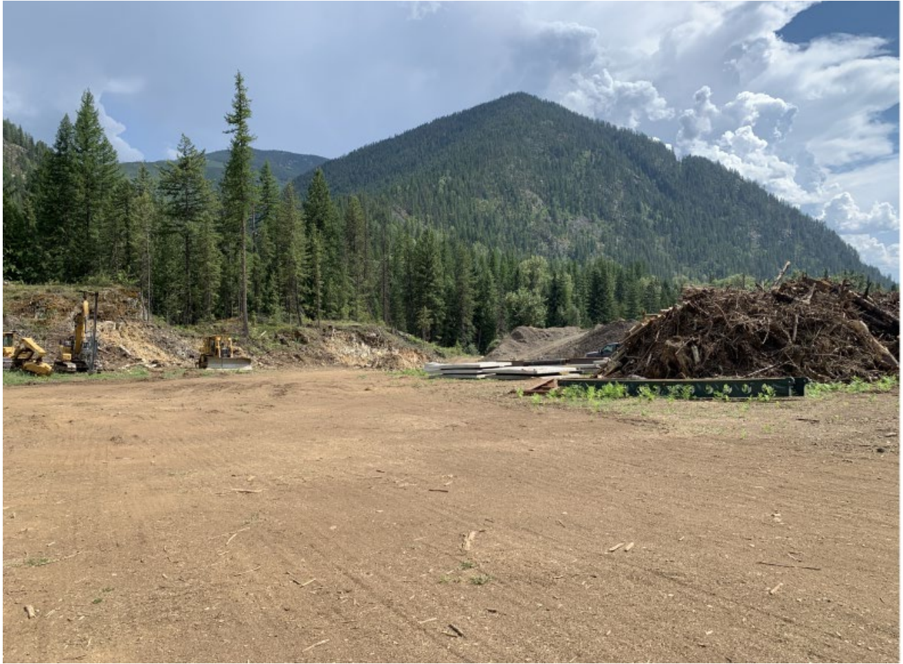
Figure 5: Subject property showing grading, earthworks and piles of trees and vegetation
