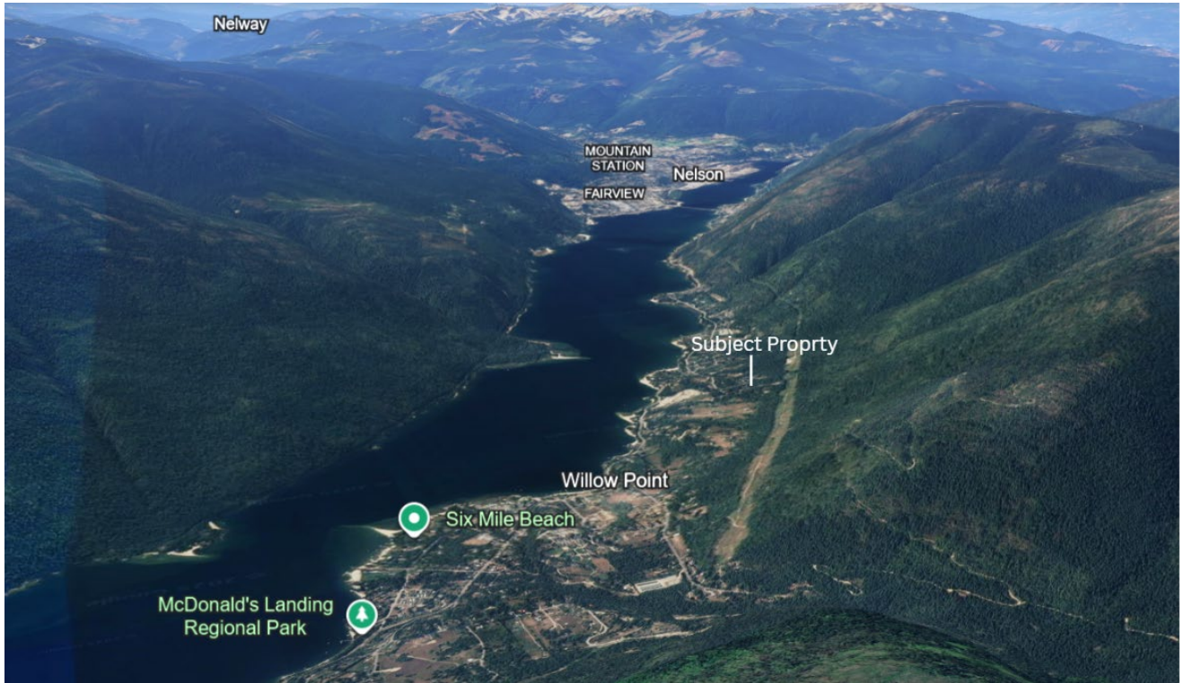
Figure 1: Context Aerial Imagery
