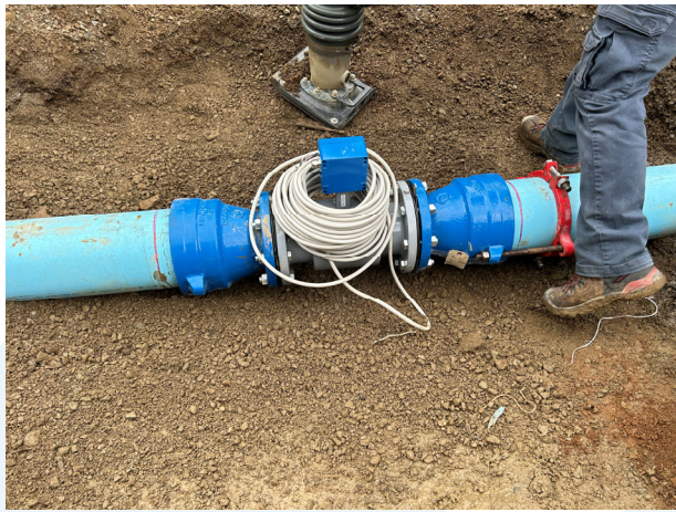
Reservoir outflow meter installation
