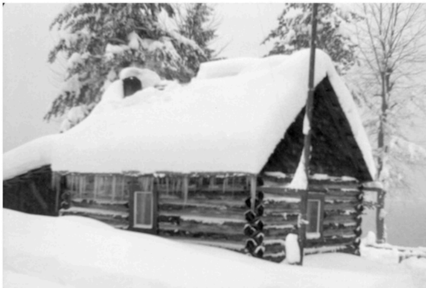
Above: Billy Clark at his cabin in the 1930s showing the door with side windows, shingled gable ends and shingled roof. Note the lack of fascia boards which were a later addition. source: BC Archives 193501-001
