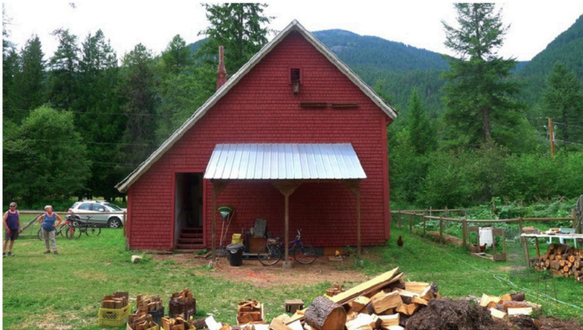
Top: Looking north east showing the lean-to extension, concrete chimney and its supports
