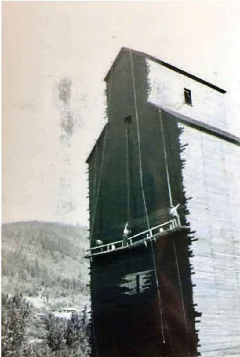
One of the elevators under construction. Creston Museum
