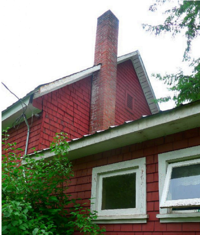
Top left: north west corner showing chimney at the intersection of the vestal and the school room, closed soffits and trim details
