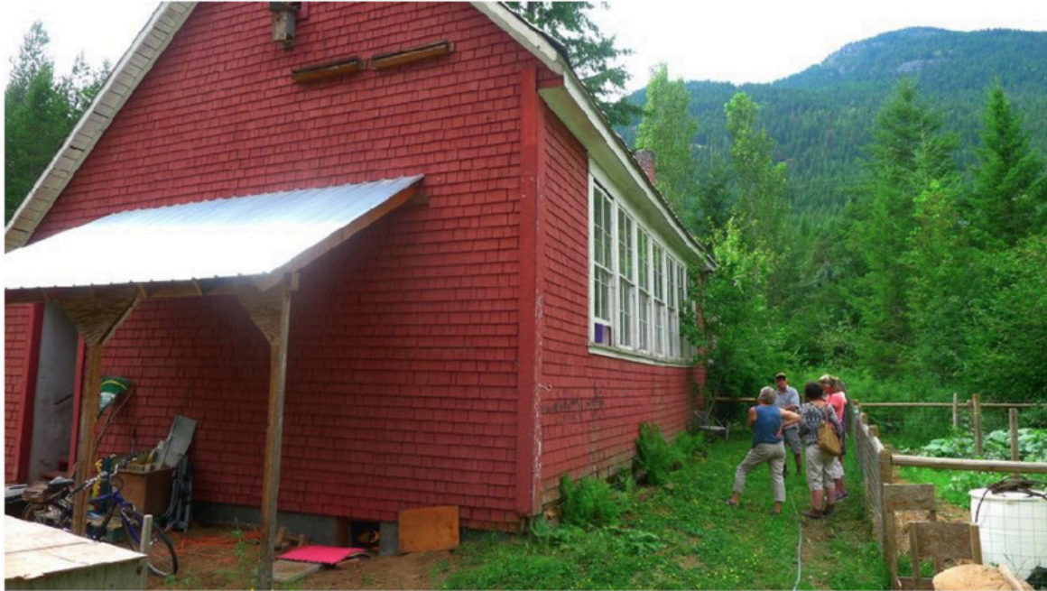
Rear and north side of the building
