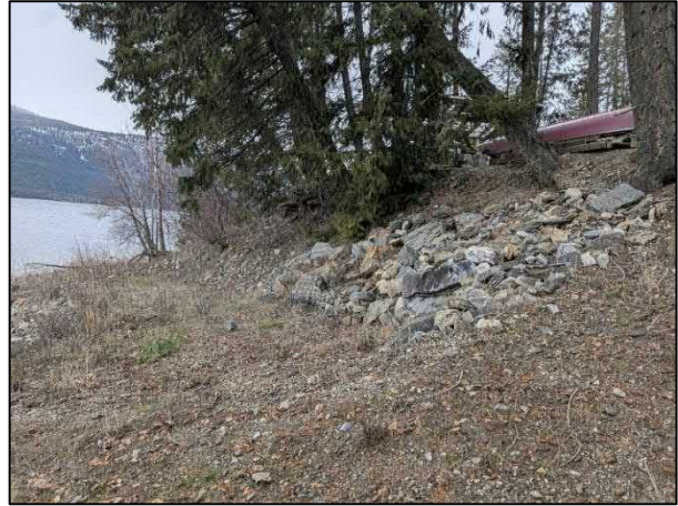
Photo 2. Erosion protection north of access road (Feb. 27, 2026).
