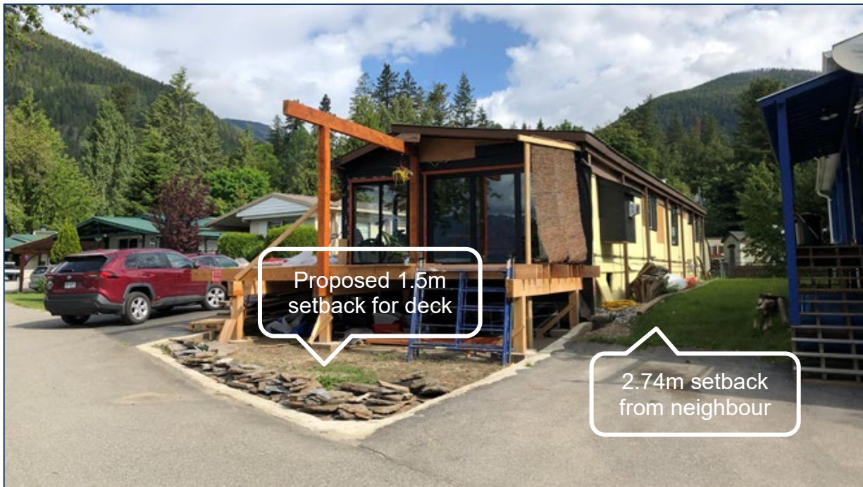
Figure 4: View of property from south-east, showing setback from front and side property lines
