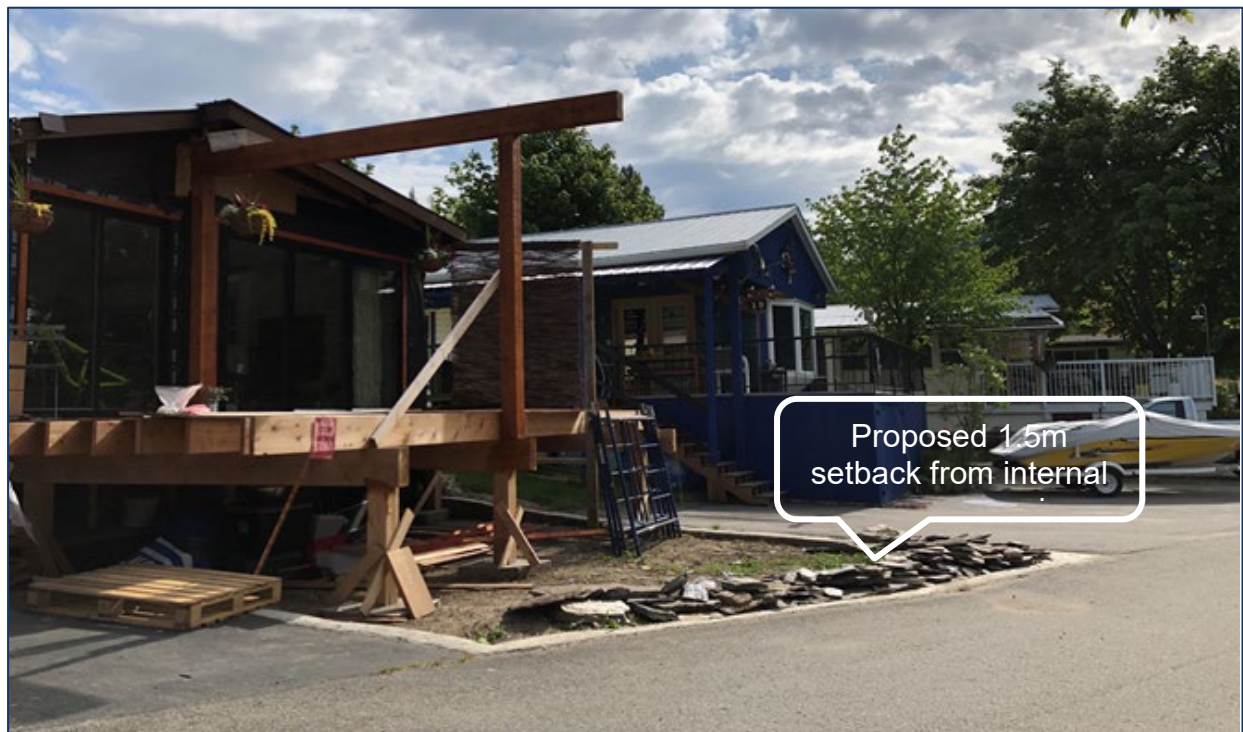
Figure 5: View of area of proposed deck as seen from the south-west
