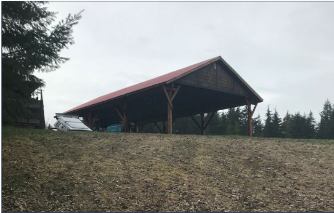
Figure 4: View of subject structure as seen from the north-east
