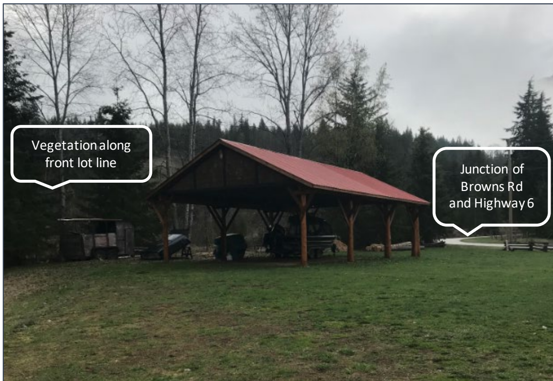
Figure 5: View of subject structure facing north-east toward the public highway
