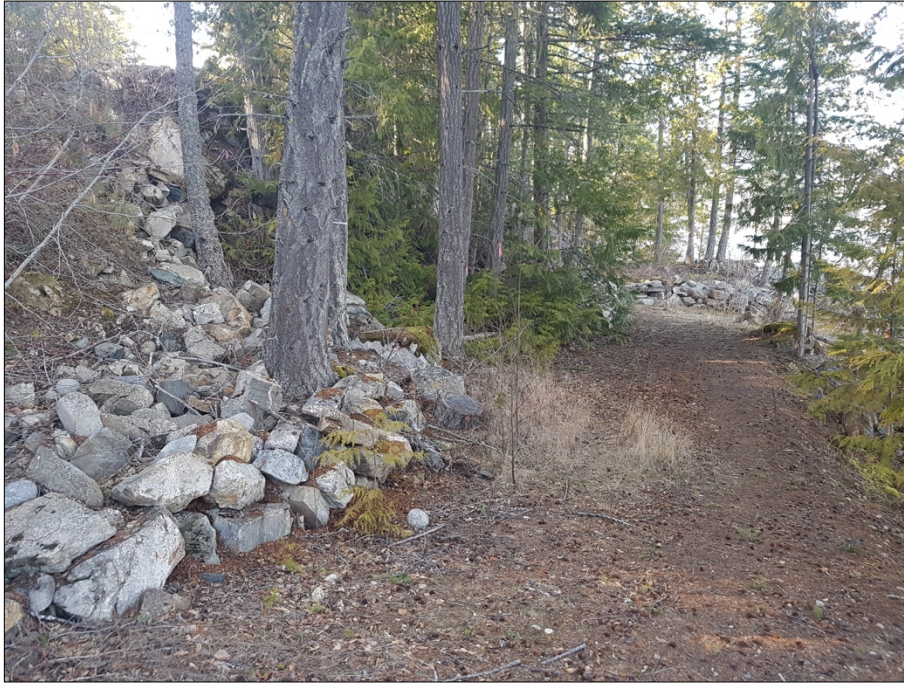
Photo 1. View northeast of the lot showing the built access road previous landscaping work undertaken as part of the preparation of the Kootenay Lake Village strata lots. Note the large talus boulders and cobbles and the steep slope talus that backs the property.
