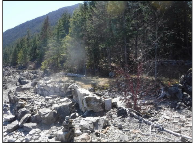
Photo 12. Tiered rock stack retaining walls supporting greenspace terrace.
