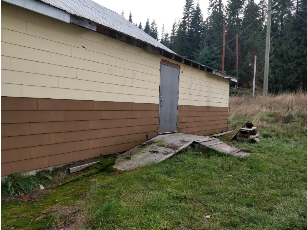
Figure 4 – Existing emergency exit does not meet current accessibility standards in the BC Building Code.
