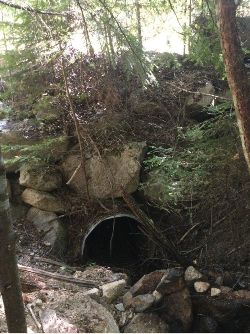
Figure 10. Private road crossing with culvert at the end of Nielson Road.
