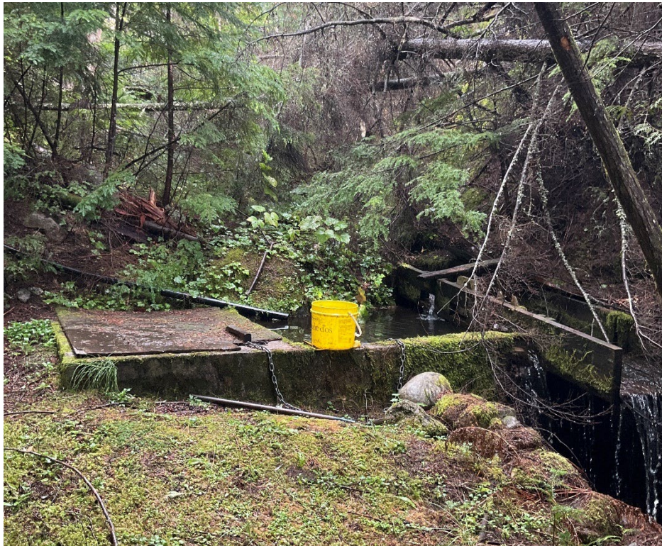
Figure 9. Water diversion structure at the apex of the Bourke Creek fan.
