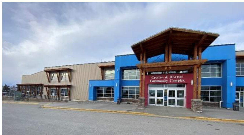
Photo 1 – Photo of facility
