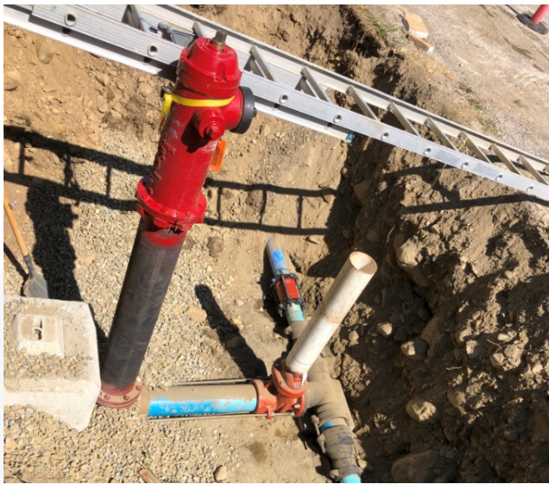
Installation of new fire hydrant in Ymir, 2022
