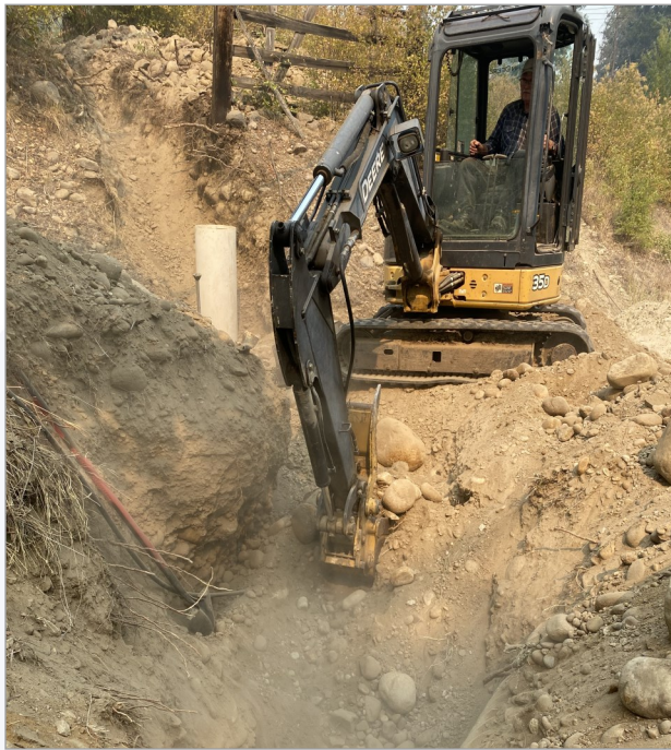
Installation of new water service on Broadwater Road
