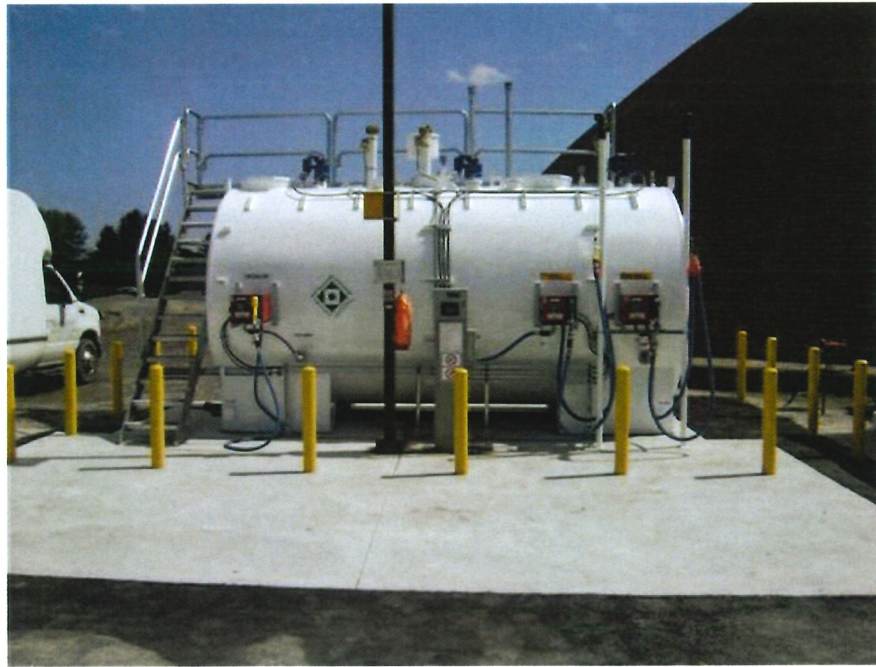
Figure 3: 25000L skidded tank example. Exact tank designed upon approval
