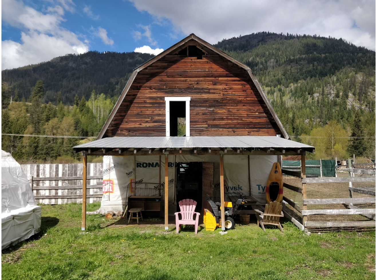
Figure 3 - Looking west at the portion of the building that is proposed to be converted to a dwelling.
